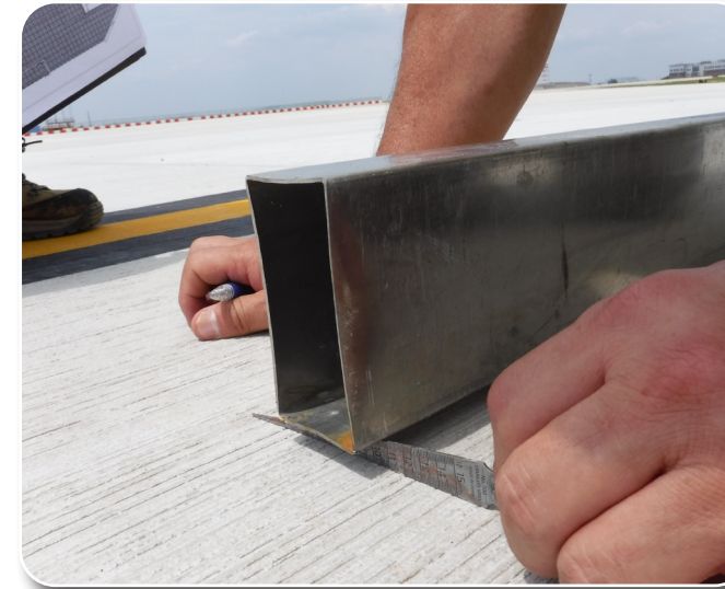
Construction Division's Quality Assurance Branch civil engineers check concrete surface smoothness on recently constructed airfield paving slabs using a straightedge.
