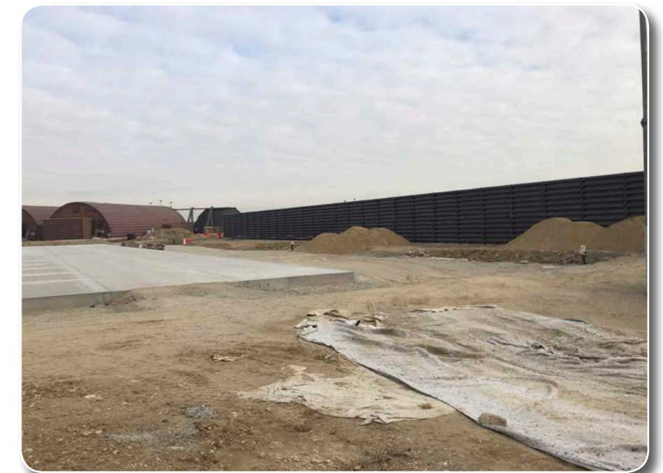
F-16 Quick Turn Pad, partially completed west pad and revetment
