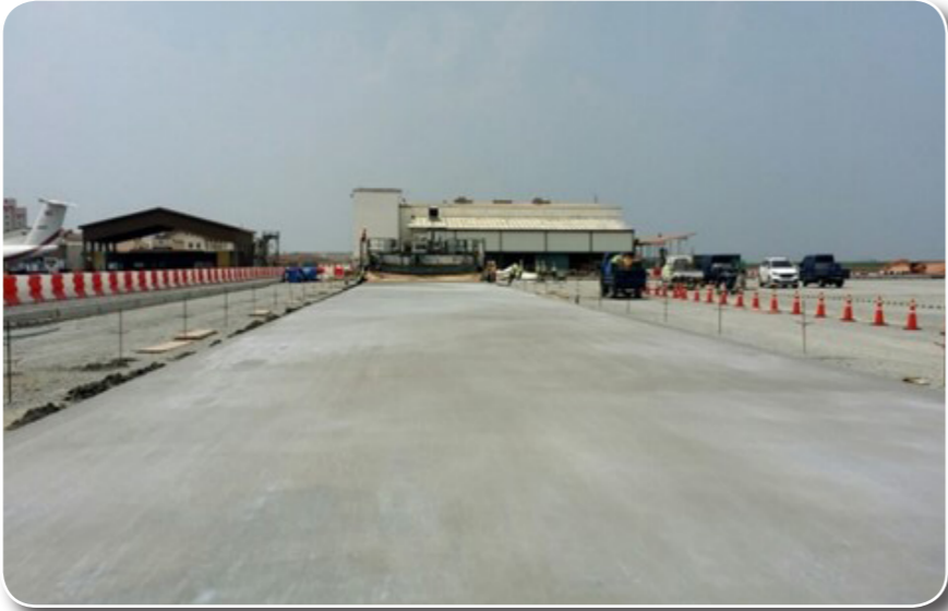
HQ050A, Aircraft Parking Apron PCC Paving
