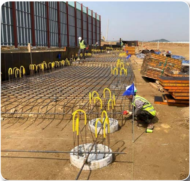
Forming rebar for retaining wall
