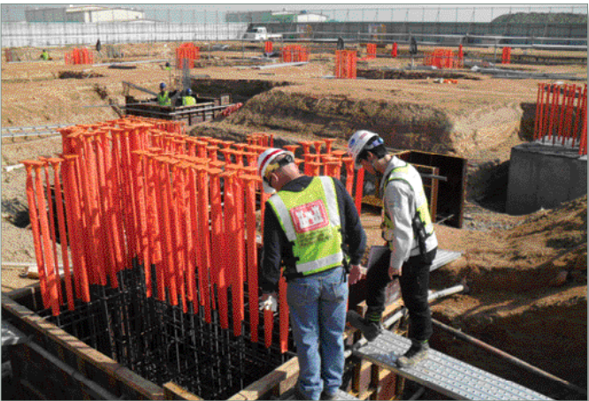
Pile cap form and rebar work
