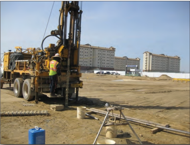
Geotechnical drilling for new facility construction in USAG Humphreys
