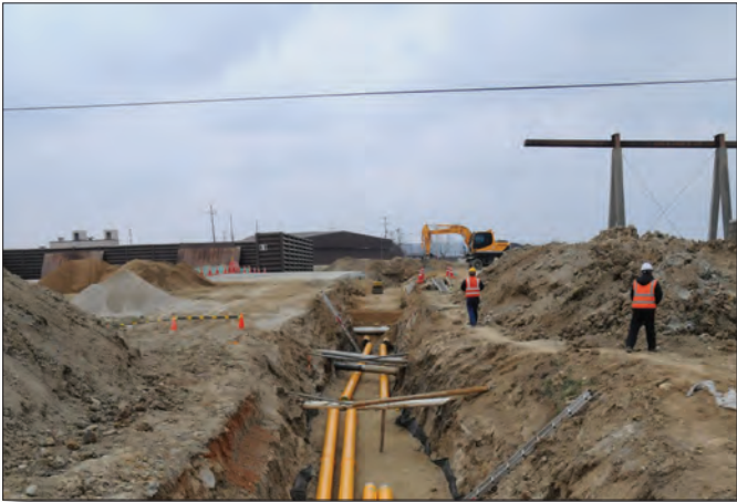
Pipe laying for fuel system
