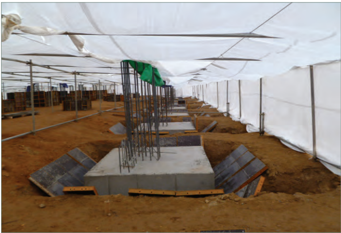
Rebar and formwork installation for pile cap
