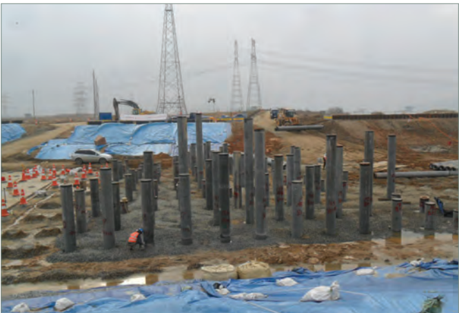
Pile Driving for Parcel 2B-2 Flood Gate Installation
