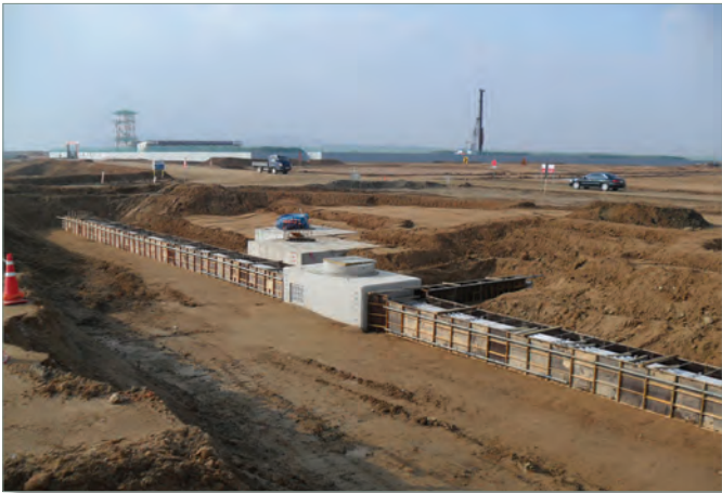
Ongoing Utility Corridor Installation in Parcel 2A
