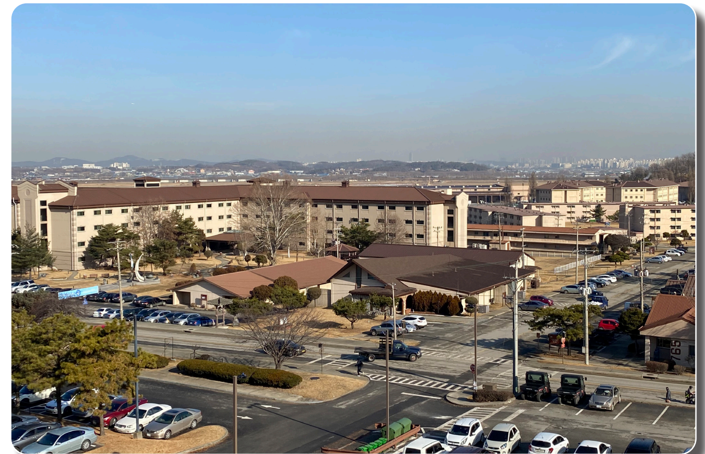
The previous, now demolished, chapel was built in 1973 and serviced about 7,000 members per month. The demolitions of the existing Chapel, Chapel Annex, and Youth Services buildings are included in the scope of work. The new Chapel is oriented at the corner of Songtan and Utah Streets with the Worship Center being the focal point of the facility. (Courtesy photo)
