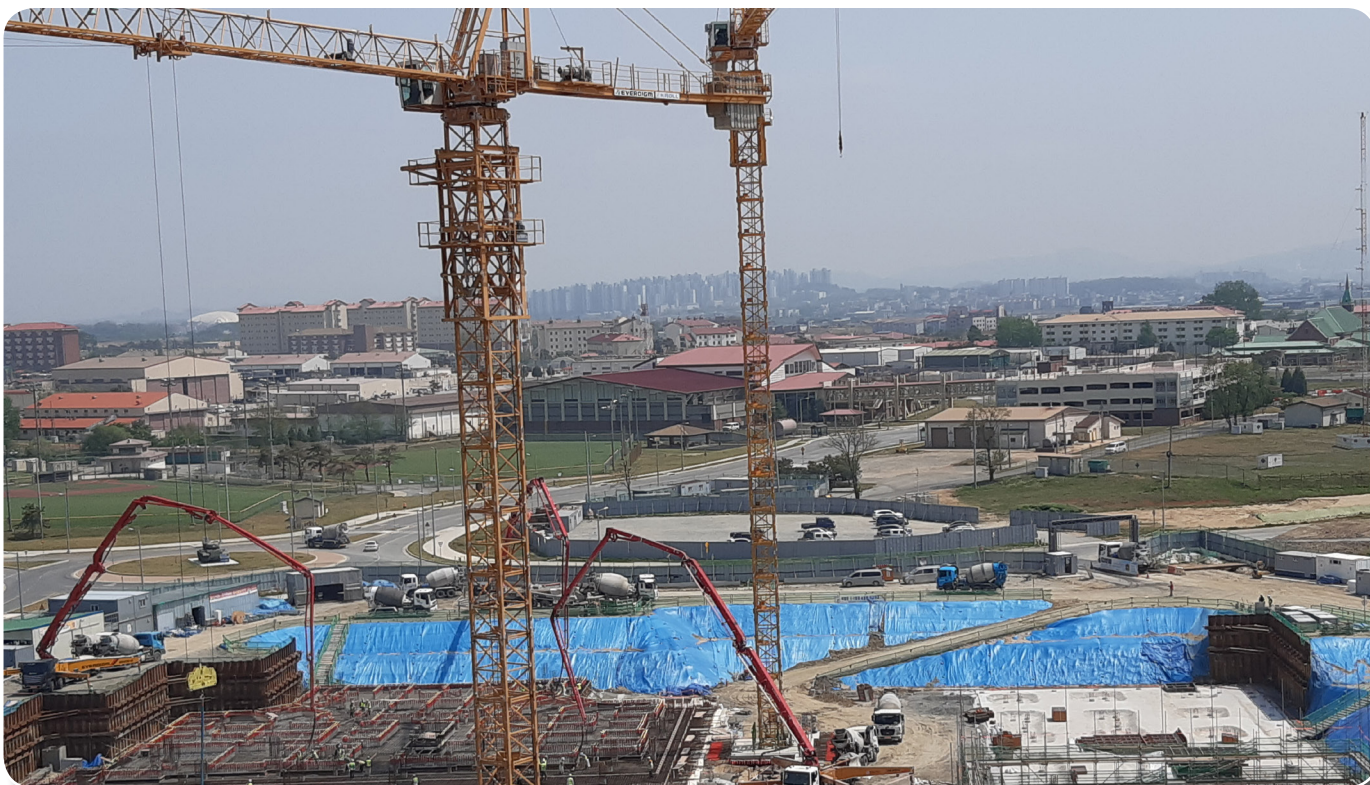
The U.S. Army Corps of Engineers, Far East District oversees a concrete placement for the AFH090 Tower 2 project at Camp Humphreys, South Korea on May 4. The towers will house senior non-commissioned officers and family members and include 144 three-bedroom units, 54 four-bedroom units, and 18 five-bedroom units. This project is scheduled to be completed by the end of 2022. (FED file photos)
