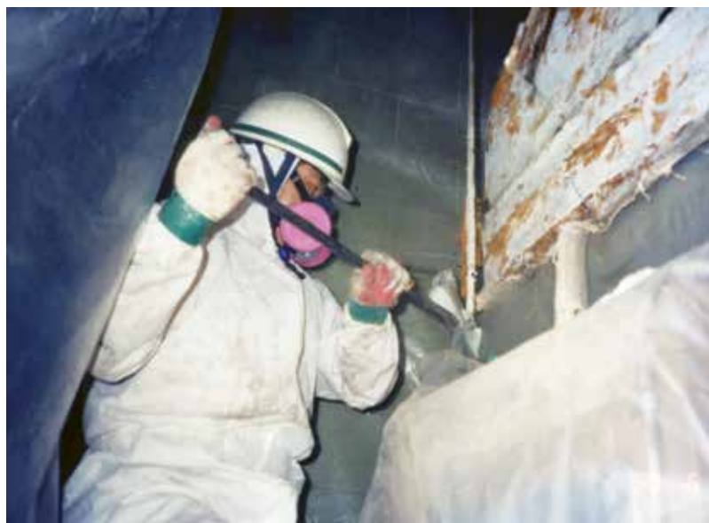
An FED contractor pries asbestos laden material from a wall in the 1990s.
