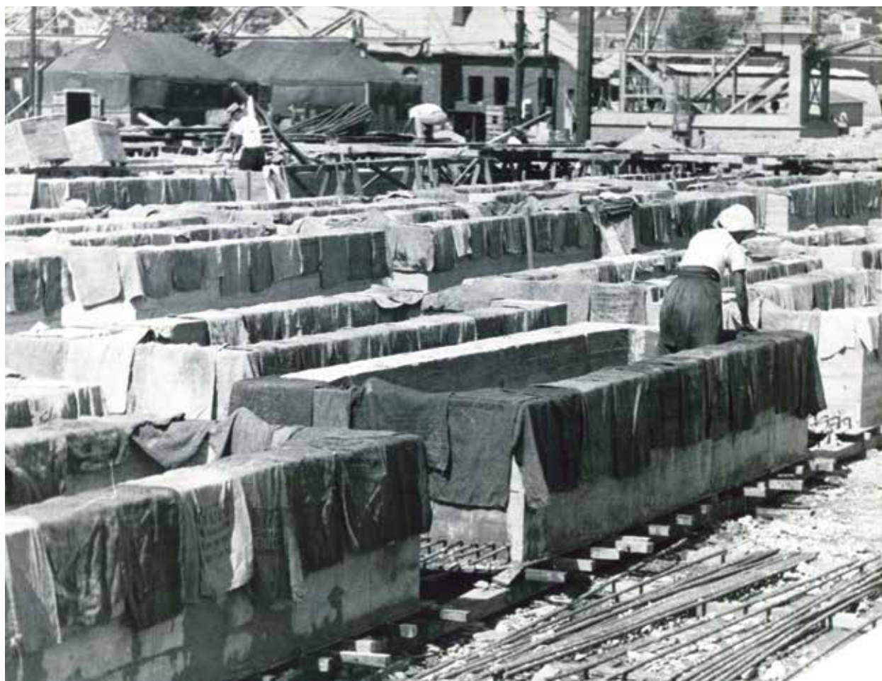
Korean workers curing the precast concrete floor beams used to repair the south wharf of the Incheon Tidal Basin, November 1959. Credit: Photo by Sergeant Ray Boswell, FED, PAO-FED Historical Files
