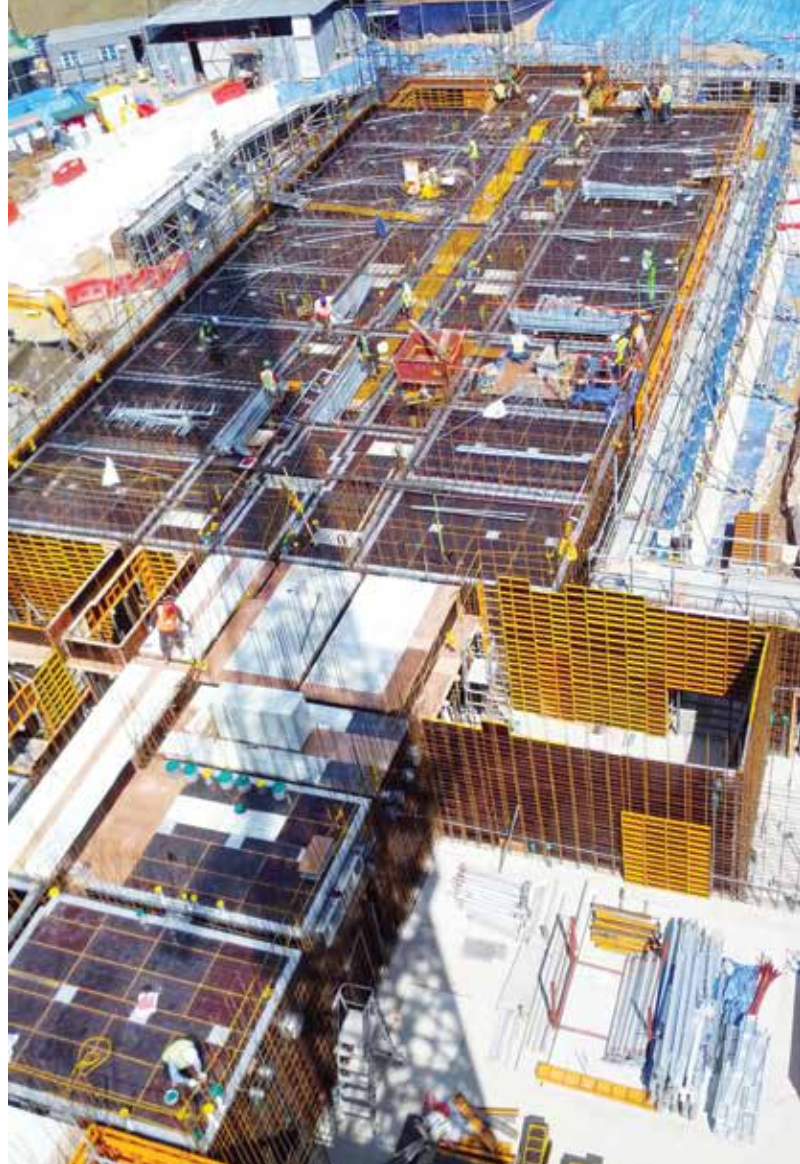
Construction of barracks at Camp Carroll using a new down slab system, 2014.
