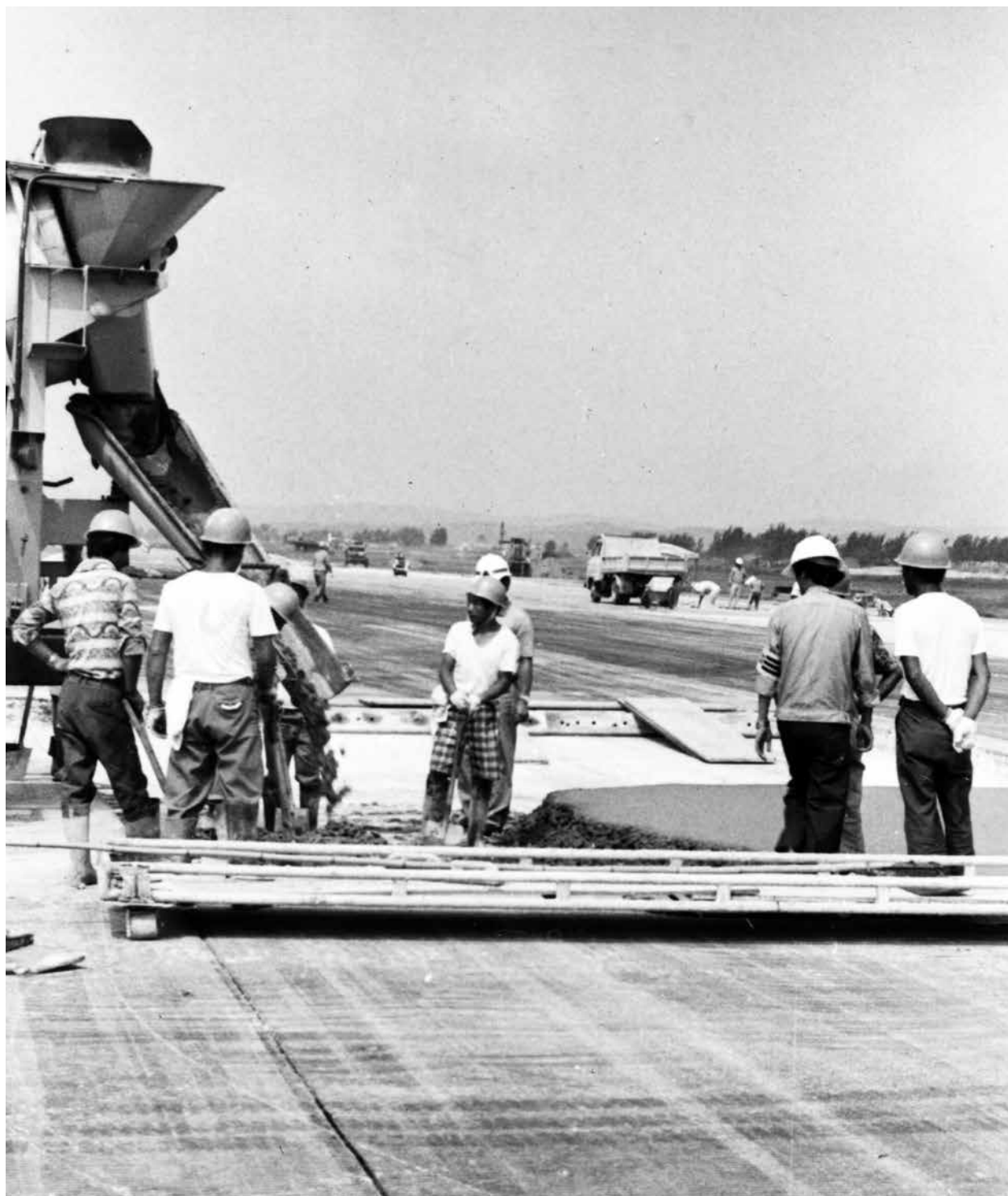
Workers for FED contractor Pum Yang pour new asphalt pavement for the runway at Osan Air Base, during the 100-day shutdown in summer 1983.
