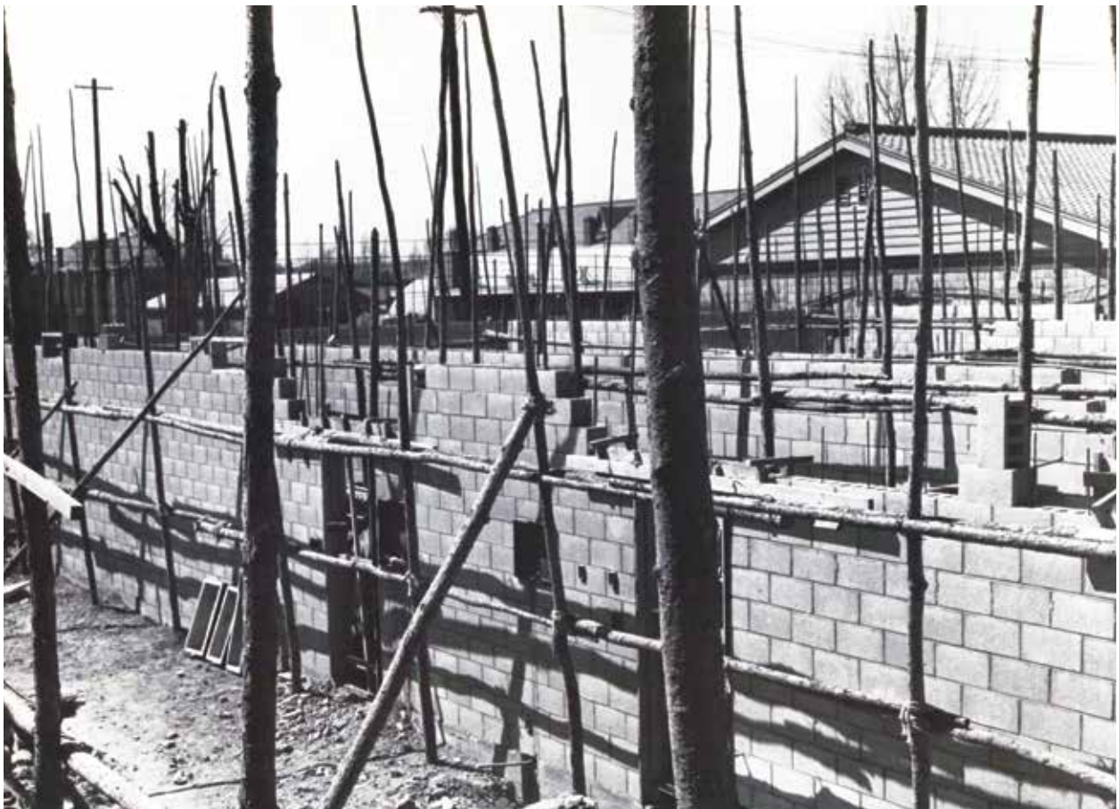
Concrete-block walls and scaffolding used to build the ACAN (Army Command Administrative Network) Communications Center, Seoul Area Command, April 1960.
