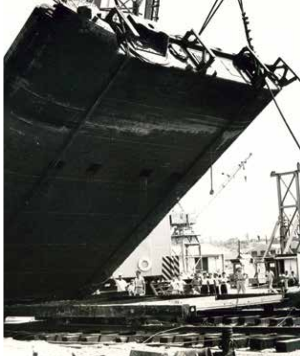
Removal of one of the 100-ton miter gates at the Incheon Tidal Basin, October 1959. Credit: Photo by Sergeant Ray Boswell, FED, PAO-FED Historical Files
