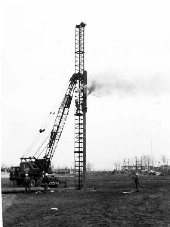
Workers using a pile driving machine during construction of troop housing at Camp Humphreys in the 1970s.
