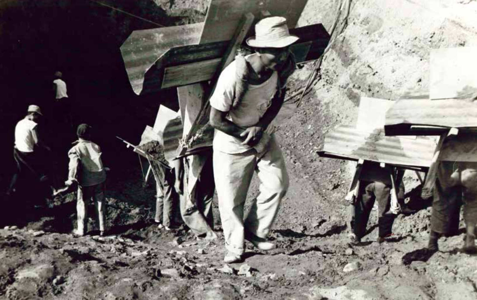
Korean laborers hauling dirt using modified A-frames, at Seoul Area Command Special Services Building, October 1960.
