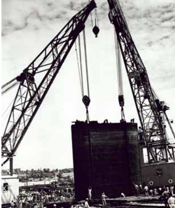
At Incheon, one of the giant leaves of the miter gate is hoisted for repair, November 1959. Credit: Photo by Sergeant Ray Boswell, FED, PAO-FED Historical Files
