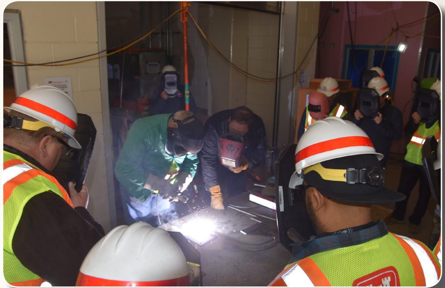
A class participant welds a piece of metal during the United States Army Corps of Engineers Far East District quality verification course March 13-17, 2017. The course teaches the participant how to interpret the various methods and techniques employed in weldments and assuring the quality of welds. (Photo by Antwaun J. Parrish)
