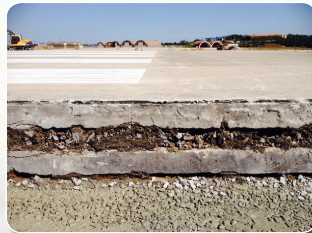
(above) An unbounded 8 inch overlay was constructed on top of the original runway in 1962. (FED file photo)
