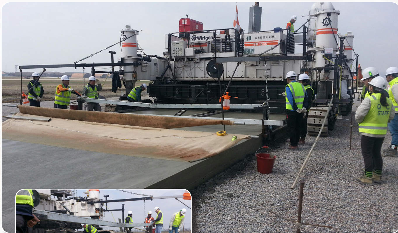
Far East District central resident office engineers and SK Engineering & Construction Co. continue to pave concrete on the 2nd runway at Osan Air Base April 7. The main runway overlay project will begin after the 2nd runway is completely paved. The pavement is to be completed by the end of 2015. (FED file photos)
