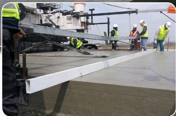
Far East District central resident office engineers and SK Engineering & Construction Co. continue to pave concrete on the 2nd runway at Osan Air Base April 7. The main runway overlay project will begin after the 2nd runway is completely paved. The pavement is to be completed by the end of 2015. (FED file photos)
