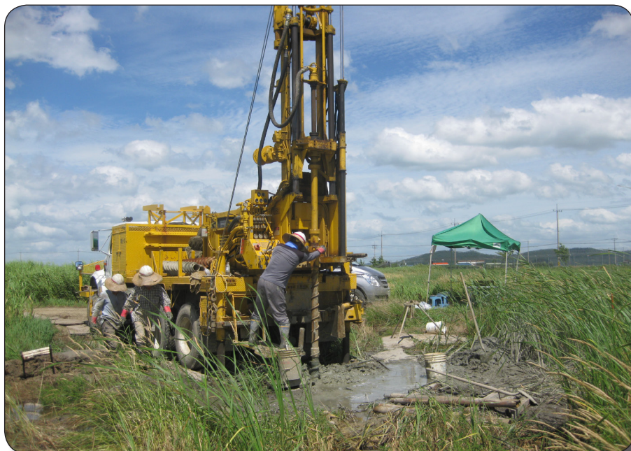
From left to right, Chang Ho-chung, Ku Chon-wan, and Yim Tok-nung of the exploration unit, geotechnical section, geotechnical and environmental engineering branch drill a borehole to test soil for the hardened aircraft shelters on Kunsan Air Base, Republic of Korea. (Photo by Pak Chung-su)
