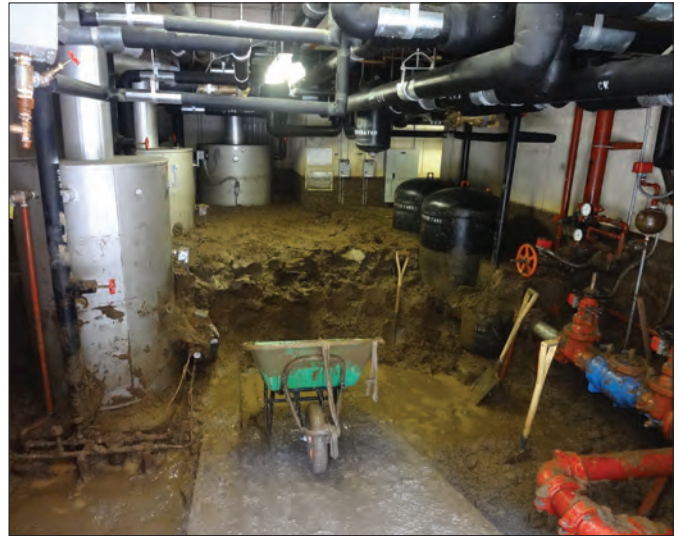
Several feet of mud buried equipment in this utility room on Camp Hovey Aug. 3 after a mudslide. The U.S. Army Corps of Engineers, Far East District Geotechnical and Environmental Engineering Branch accessed the damage in Area I in the following days. (FED File Photo)
