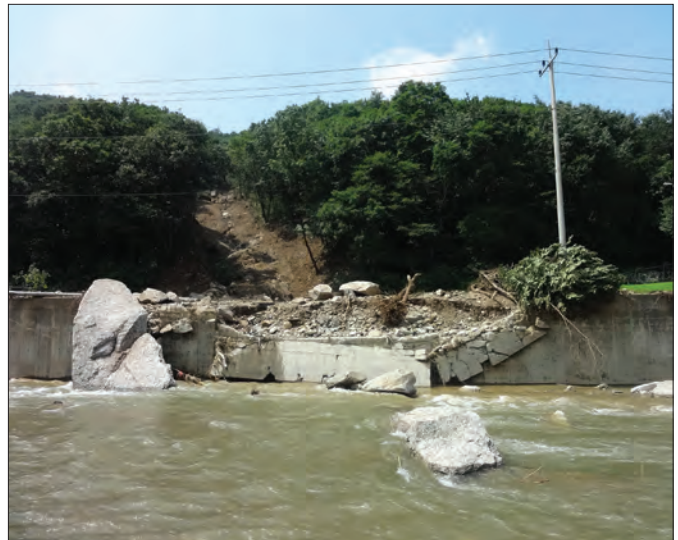
A section of the wall which forms the channel flowing through Camp Casey and Camp Hovey was washed away by a mudslide Aug. 3. The U.S. Army Corps of Engineers, Far East District Geotechnical and Environmental Engineering Branch accessed the damage in Area I in the following days. (FED File Photo)
