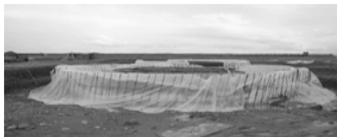
Two water tank foundations for the water treatment plant with two footers placed
