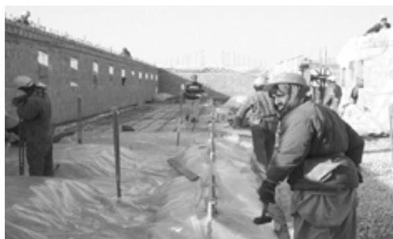
Preparing a barracks for the concrete floor
