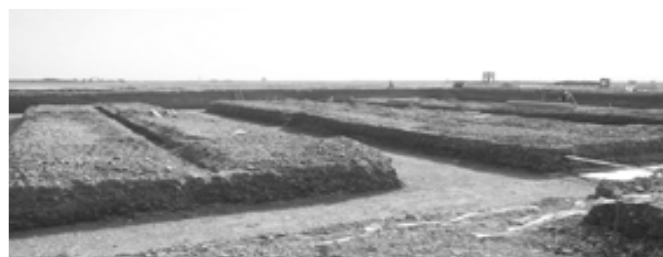
Excavation for the drying beds for the waste water treatment plant
