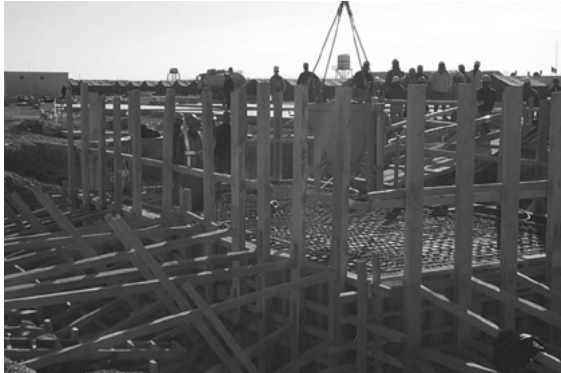
Concrete being placed 1.5 cubic meters at a time
