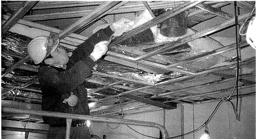
(Above) Construction worker installs insulation in the ceiling of Building S-81, during the renovation for the new crisis management center. (Below) The new emergency operations center in Seoul is in action during the RSOI exercise.
