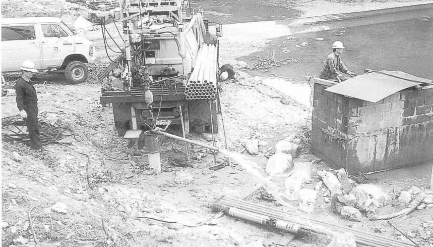
(above left) The Foundation and Materials Branch well maintenance team flushes water from well 24 at Camp Hovey and cleans the pipes removed from the well. (above right) Doug Bliss, Chief, Foundations and Materials Branch, FED, is interviewed by AFKN television about the well maintenance and repairs.
