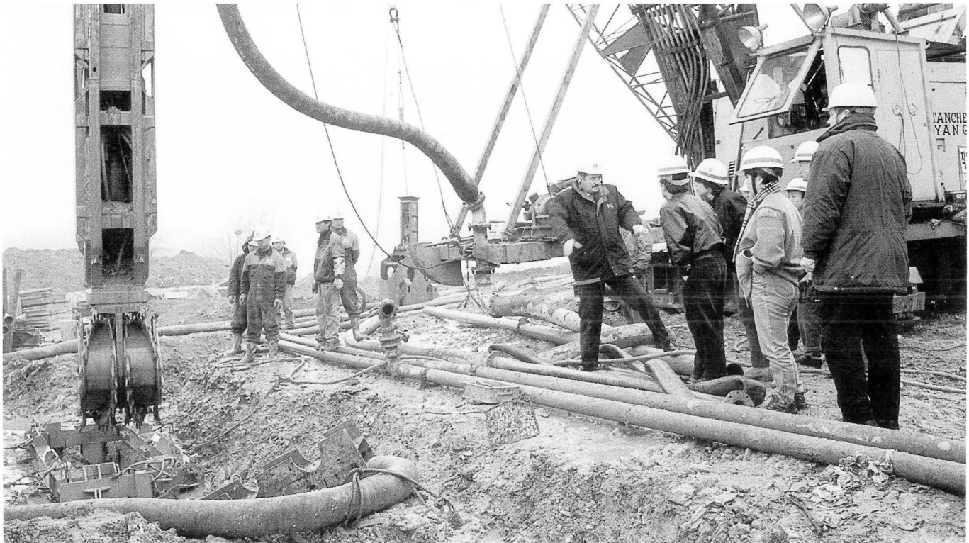
On Friday, February 27, FEDsters toured the Nangido Landfill Construction site. Construction has begun on a combination cement bentonite slurry wall and sheet pile wall which will encircle the landfill. The slurry wall will be 3,320 meters long, 800 millimeters high and approximately 3 feet thick and include 31 pumping wells and 45 gas wells.
