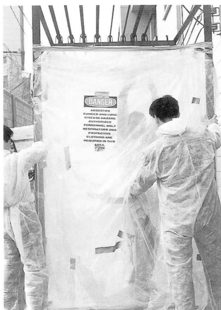
abatement containment and decontamination (decon) chamber.
