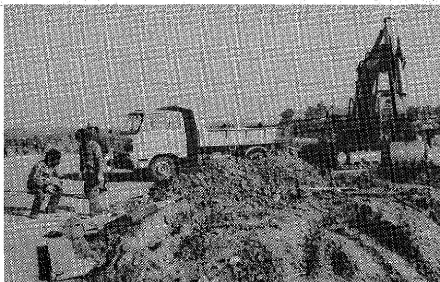
FED contractor personnel are shown at work at Osan Air Base in October 1983. They are constructing a new overrun area for the runway, part of the $6.7 million repair and improvement job there. This critical Air Force project was successfully completed through good FED-AF cooperation.
