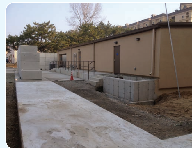
Demolition/Consolidation of B511/512
