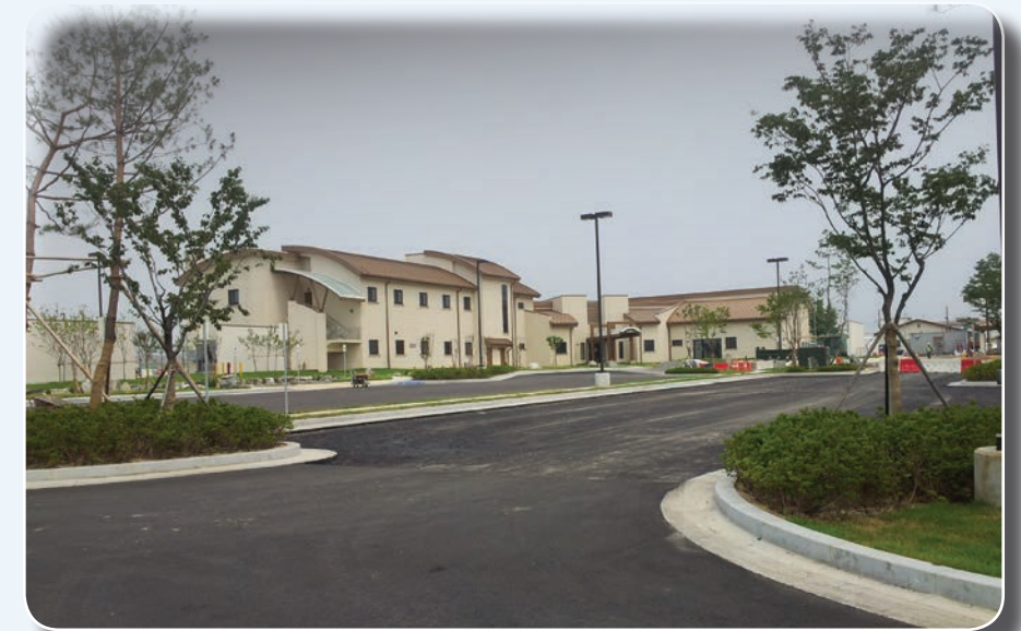
Airfield operations building
