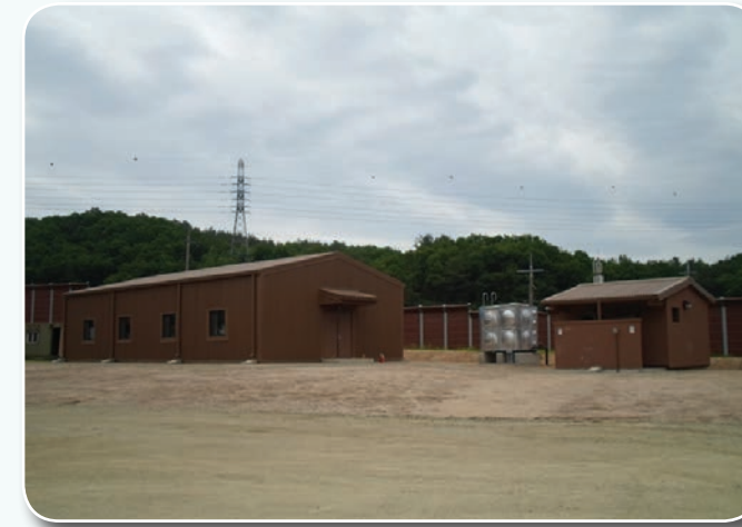
New Facility, Warrior Valley Range
