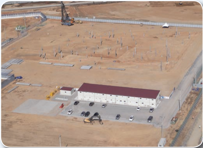
U.S. Korea Command Headquarters – Pile driving
