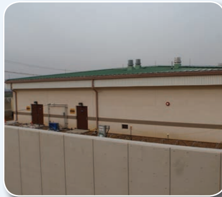
ADN building 93 percent completion
