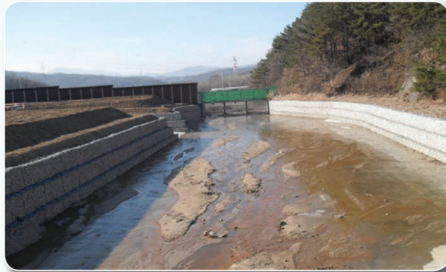
Drainage, Warrior Valley Range
