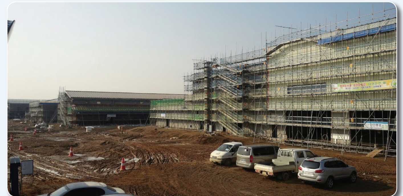
CY11 HBCT Vehicle Maintenance Facility I
