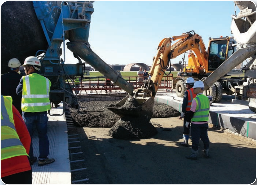
Repair of main runway
