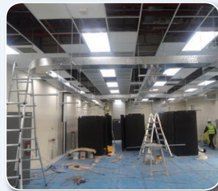
Server room under construction
