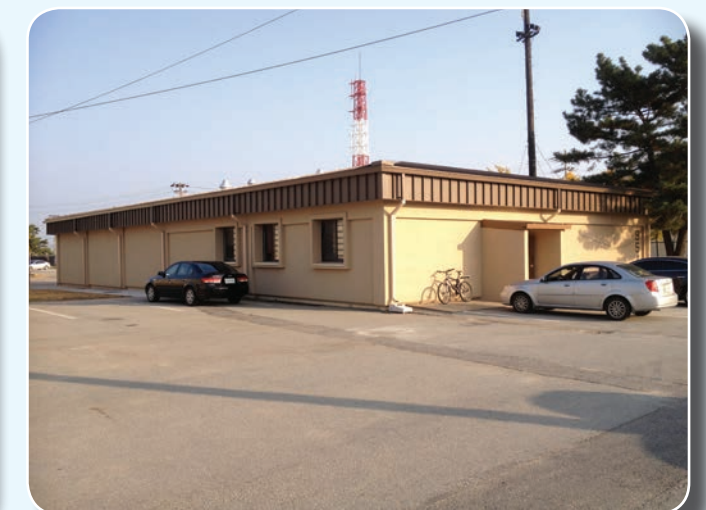
Demolition/Consolidation of B950/954
