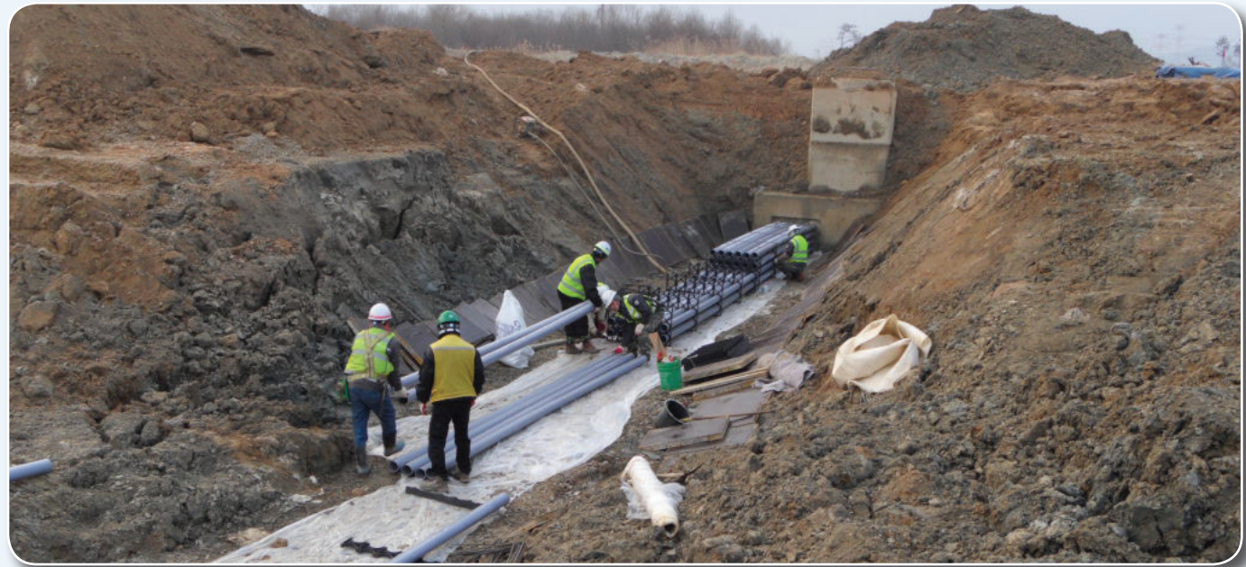
Constructing C4I duct bank
