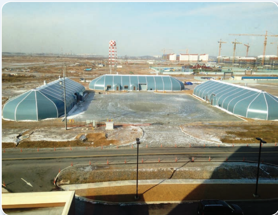
Televideo Center and Swing Space
