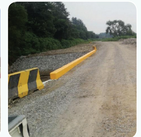
Repair and Upgrade of Maneuver Trail #1, Dagmar-North
