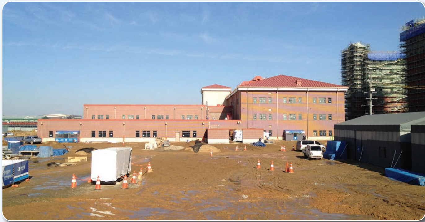
CY10 HBCT Consolidated Headquarters
