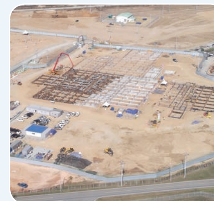
CY08 YRP Eighth Army/CNRK Headquarters – Concrete beams
