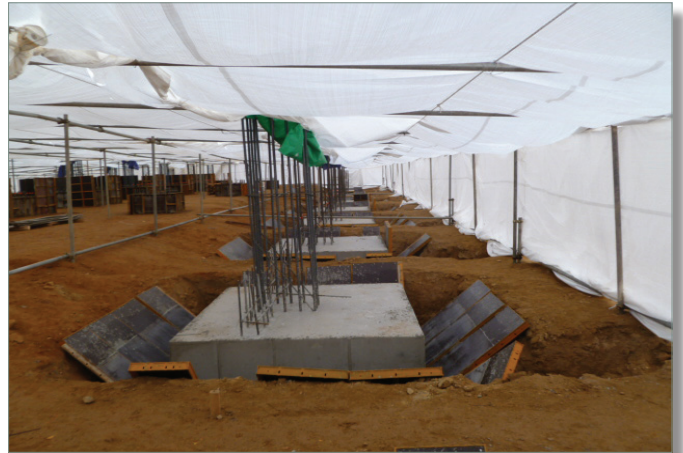
Rebar and formwork installation for pile cap
