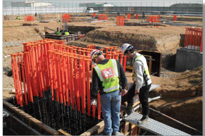
Pile cap form and rebar work
