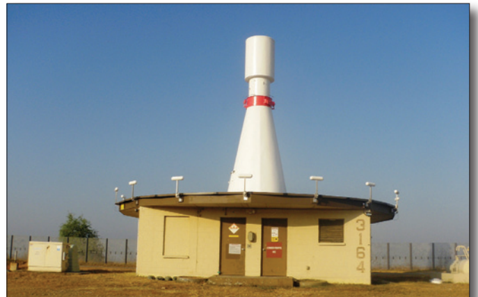
VORTAC radar roof replacement
