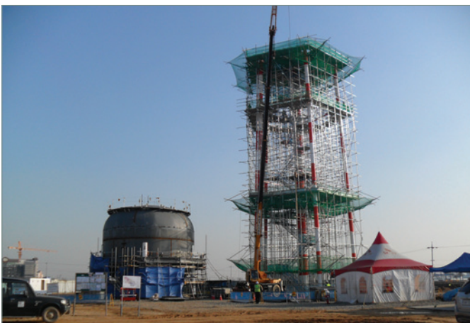
250,000 Gallon Elevated Water Storage Tank
