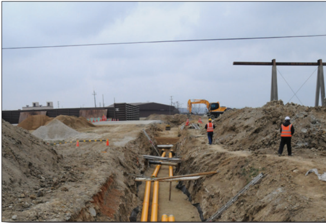
Pipe laying for fuel system
