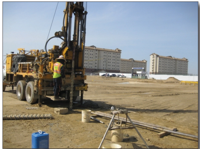
Geotechnical drilling for new facility construction in USAG Humphreys
