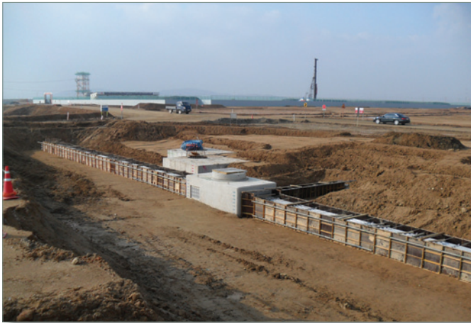
Ongoing Utility Corridor Installation in Parcel 2A
