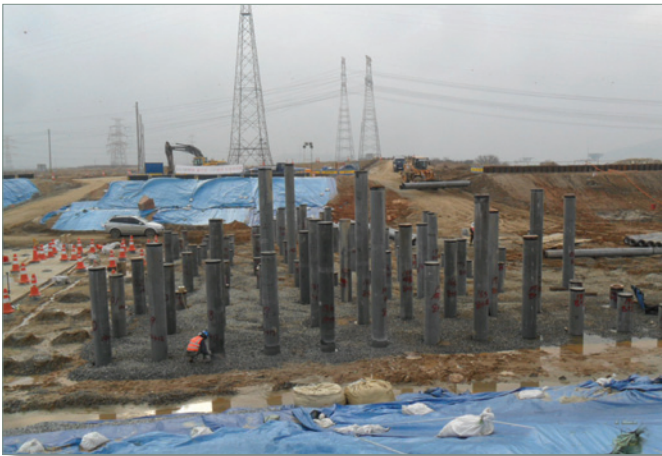
Pile Driving for Parcel 2B-2 Flood Gate Installation
