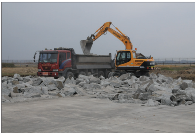
Removing old concrete for a new hot cargo pad
