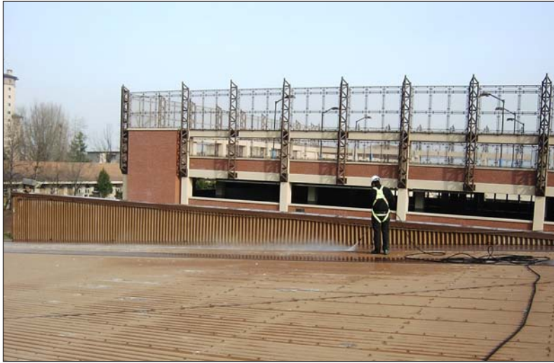
EPDM roofing commissary cleaning by pressure water
