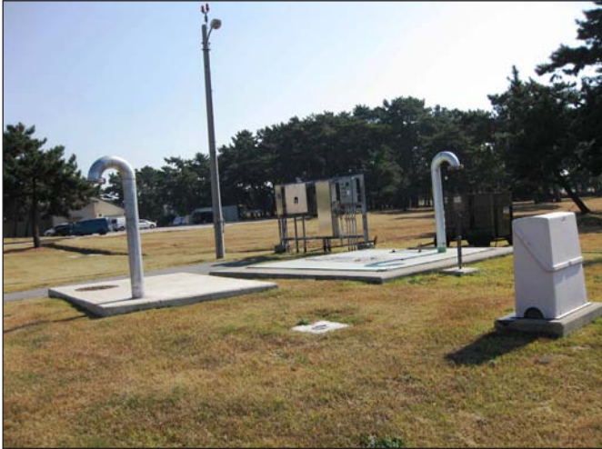
Upgraded Sewer Lift Station
