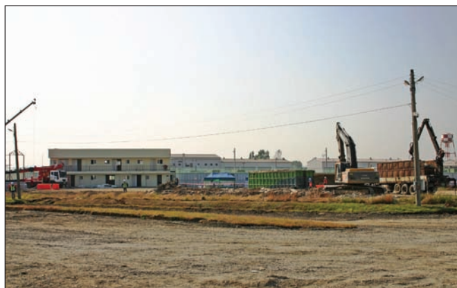
Clearing and grubbing work at FY10 Fire Station site
