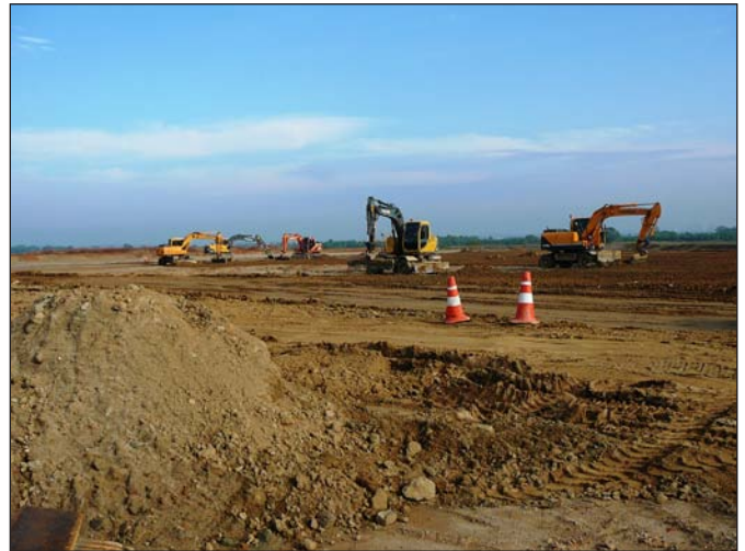
Placement of engineering backfill material in Parcel 2A
