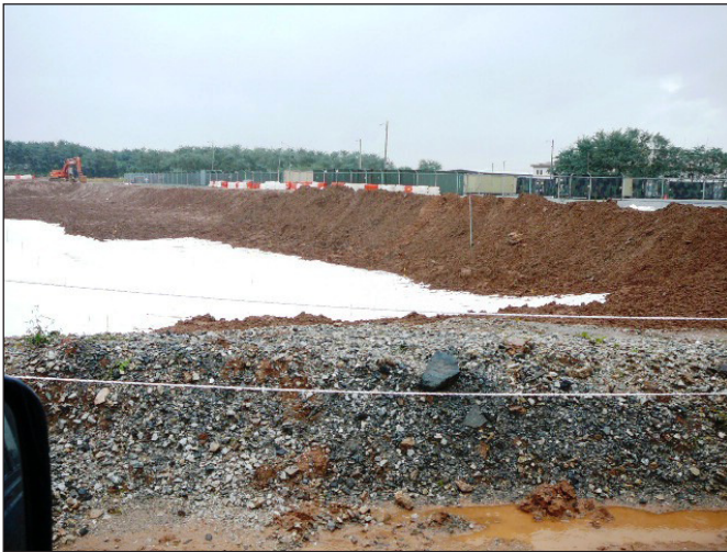
Installation of geotextile
