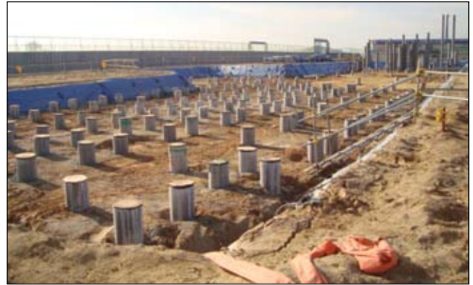
Piles for FY07-08 MCA Barracks Complexes
