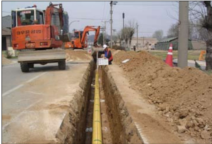
Installing Gas line, K-16
