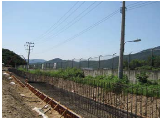
Form and rebar work for Noise Abatement Wall Foundation
