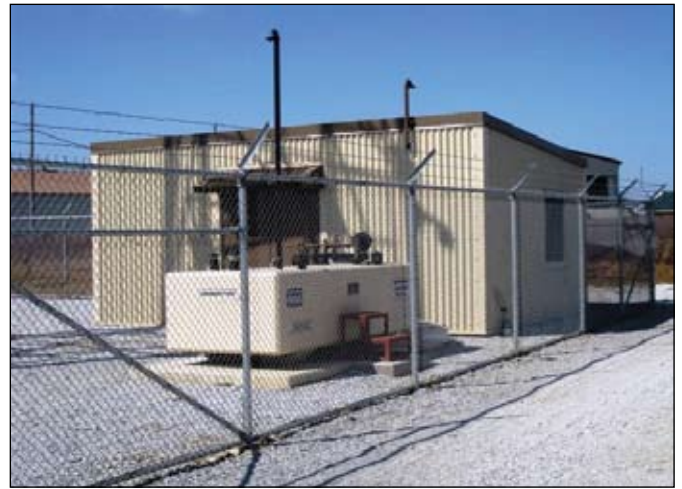
Generator and Fuel Storage Tank
