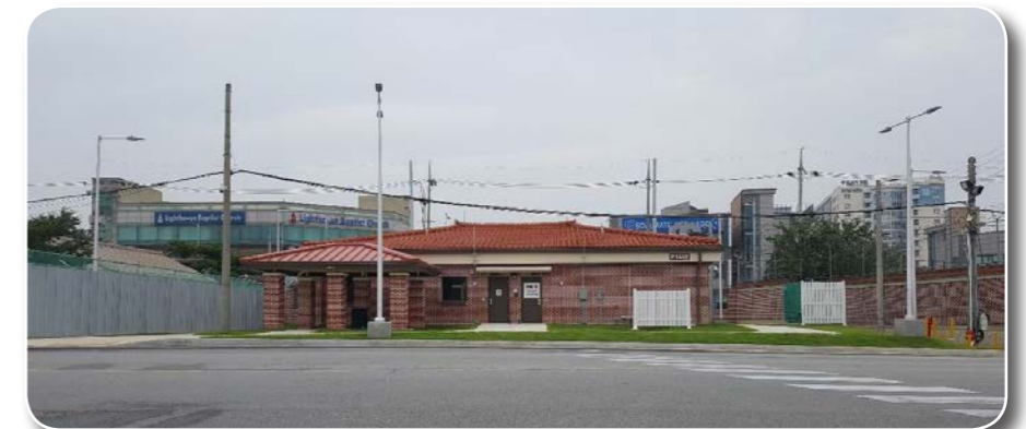
VCC010 Visitor Control Center - Pedestrian Gate
