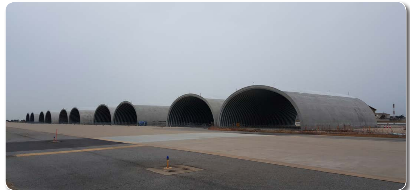
Hardened Aircraft Flow Thru Shelter
