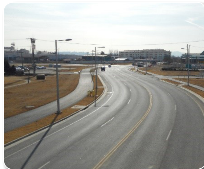
Land Development and Utilities Infrastructure, Parcel 2A and Existing Humphreys
