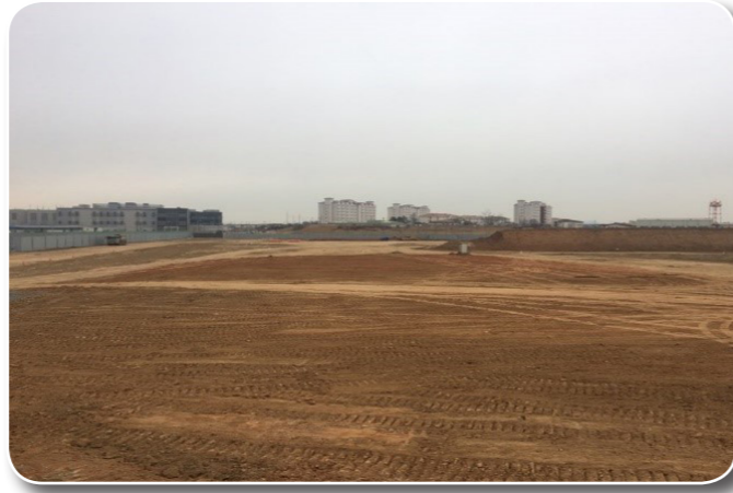
AFH100 Family Housing New Construction site
