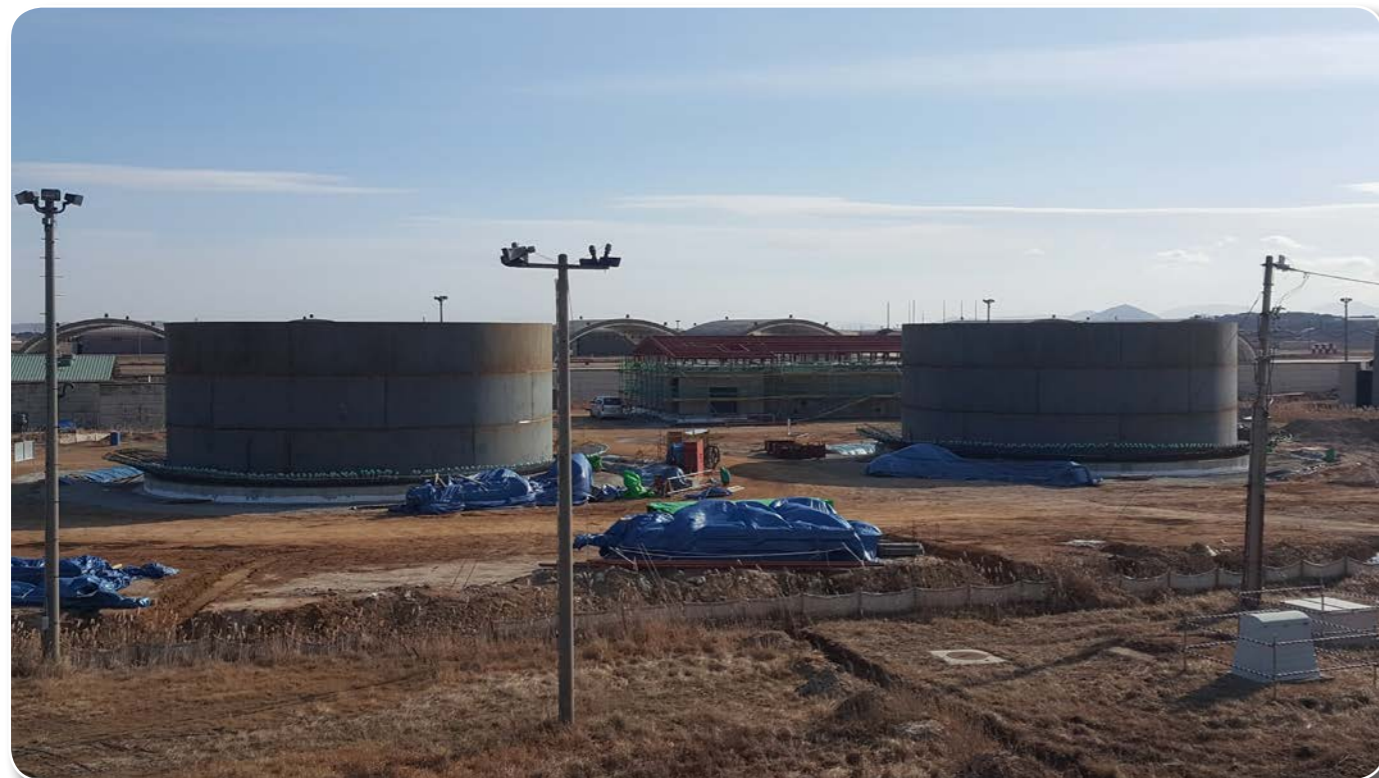
Hardened Aircraft Flow Thru Shelter
