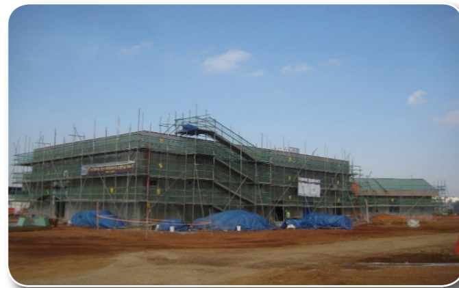
MWR Restaurant Construction Ongoing
