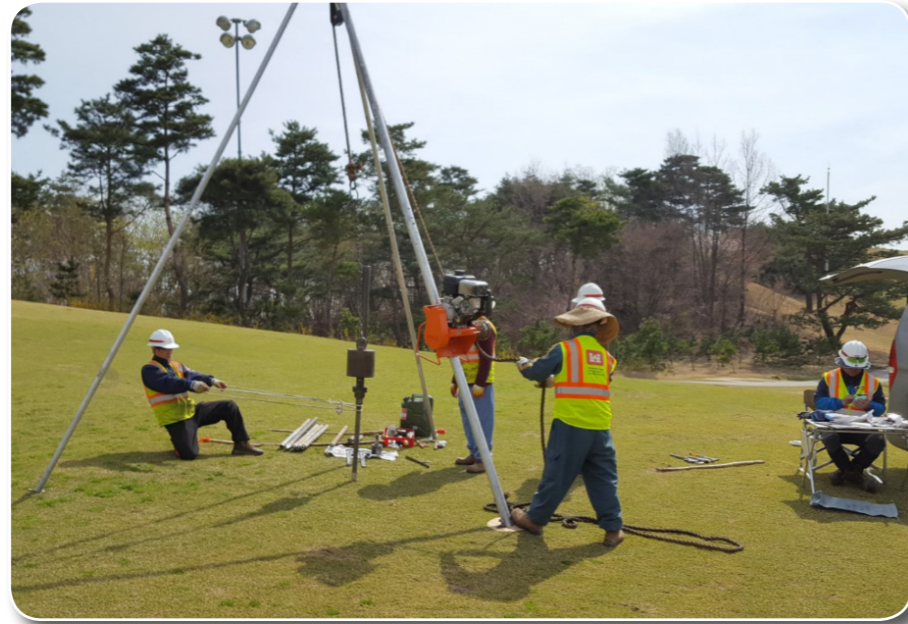
Soil Boring for THAAD Deployment Korea Project
