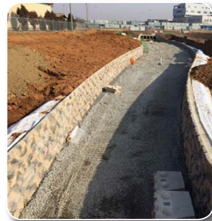
Repair of Storm Drainage
