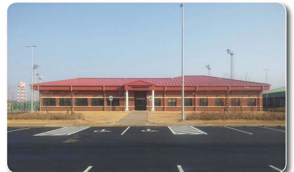
Early Development and Intervention Services (EDIS) Facility
