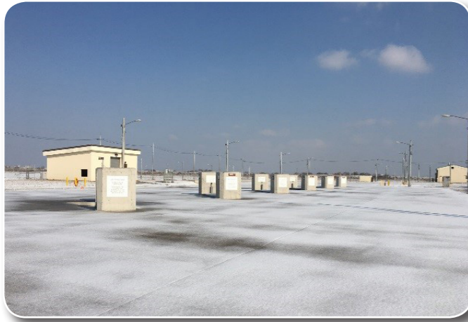
Pump House and Tank Wash Stations
