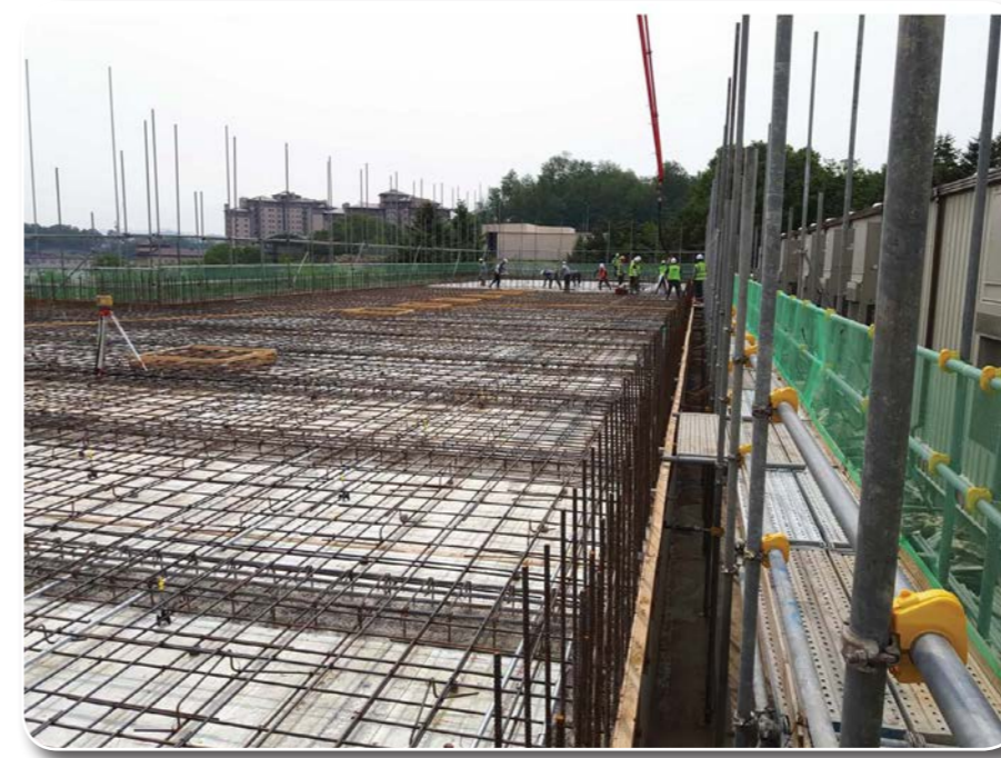
694 ISRG Secure Storage Facilities
