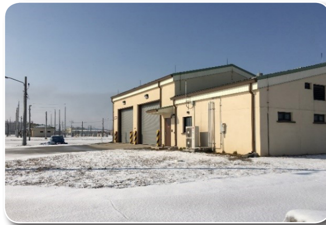
Vehicle Maintenance Bay
