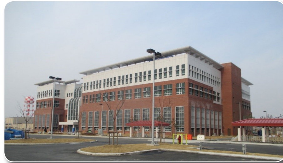
HQ050 Site#1 Far East District Headquarters Building
