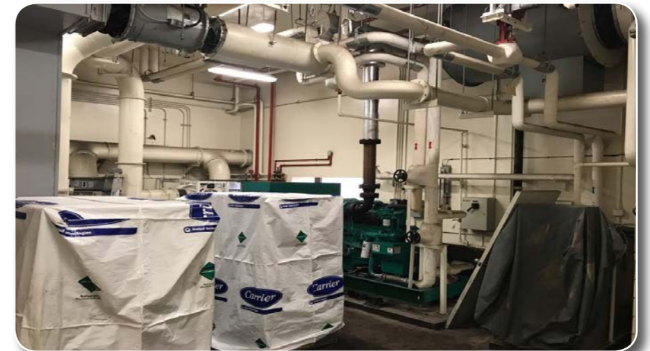
HVAC Repair/Replacement Task Order #0079
