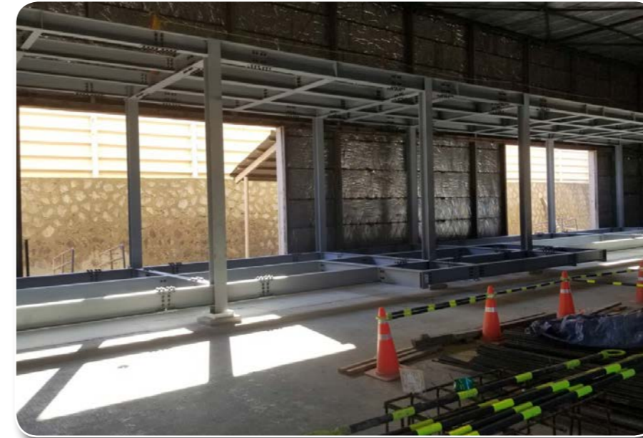
VIP Hangar and Parking Pads
