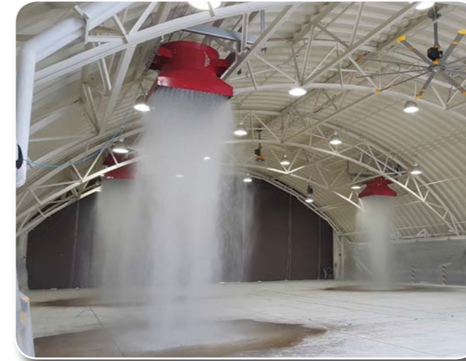
Repair of Fire Protection System for Hangar 1729
