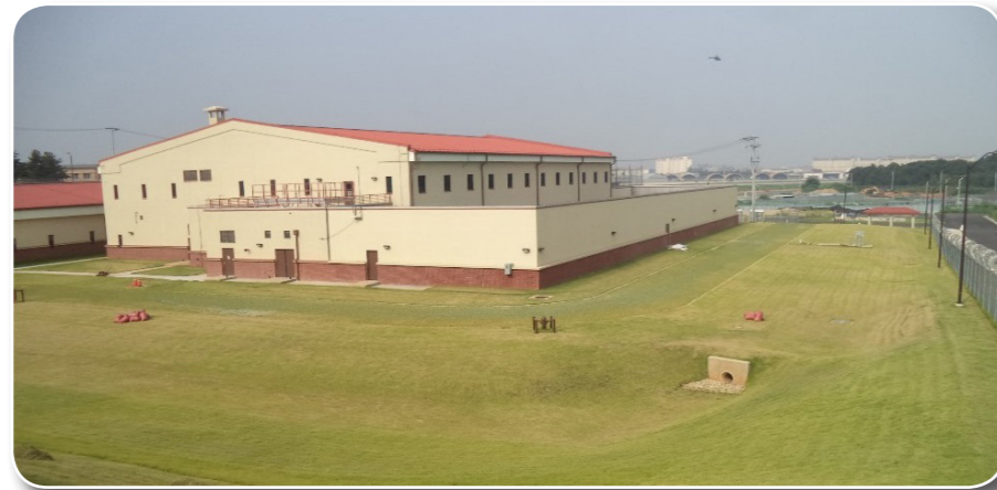
UEH20B 501st Brigade Headquarters Building
