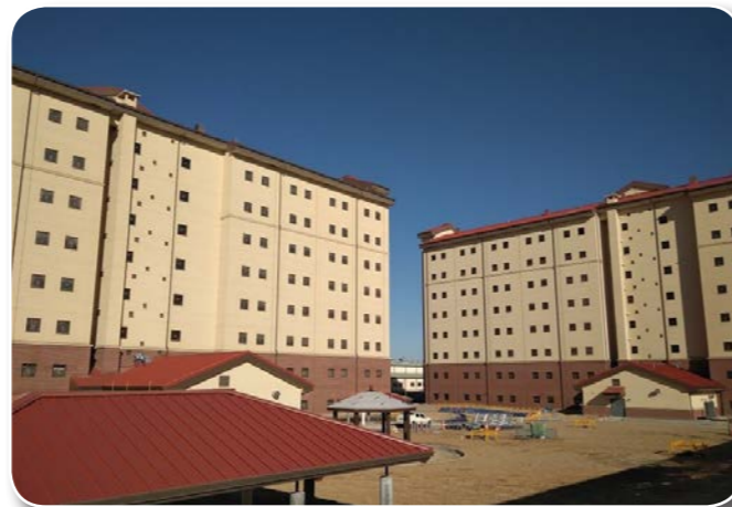
UEH050 Unaccompanied Enlisted Personnel Housing
