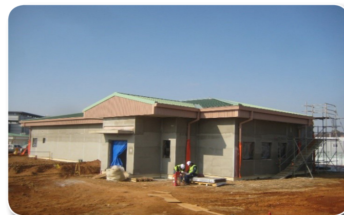
KATUSA Snack Bar Construction Ongoing
