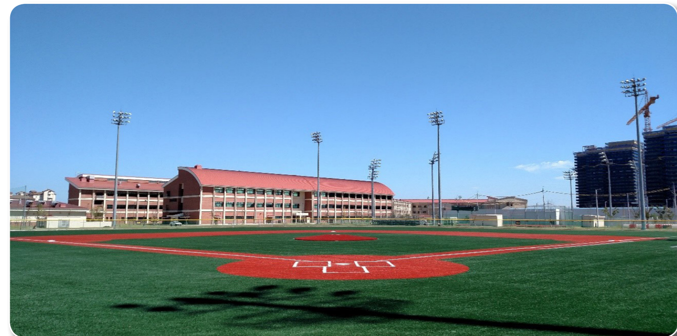
Repair of Current Softball and Baseball Field at High School
