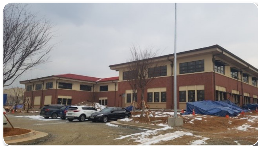
C41050 Administration Building
