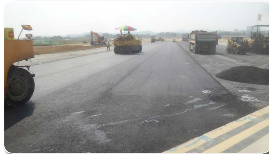
Main Runway Repair
