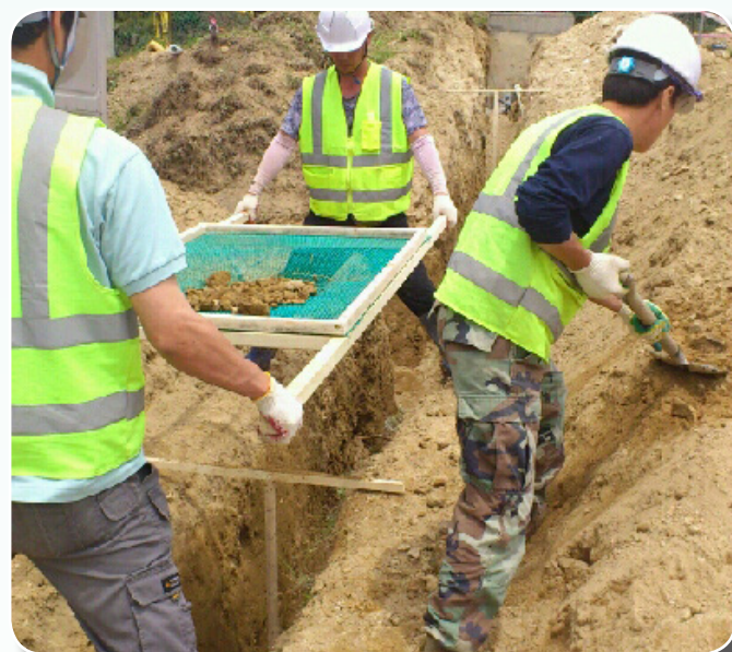
Water pipe replacement at Camp Madison
