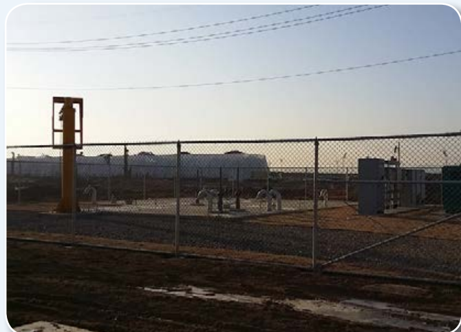
Lift Station #8 at the corner of 9th and E-Avenue
