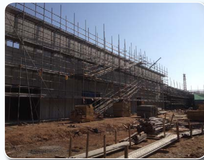
CY13 ROKFC-in-Kind, Communication Squadron Facility
