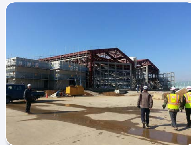
Aircraft Corrosion Control Facility
