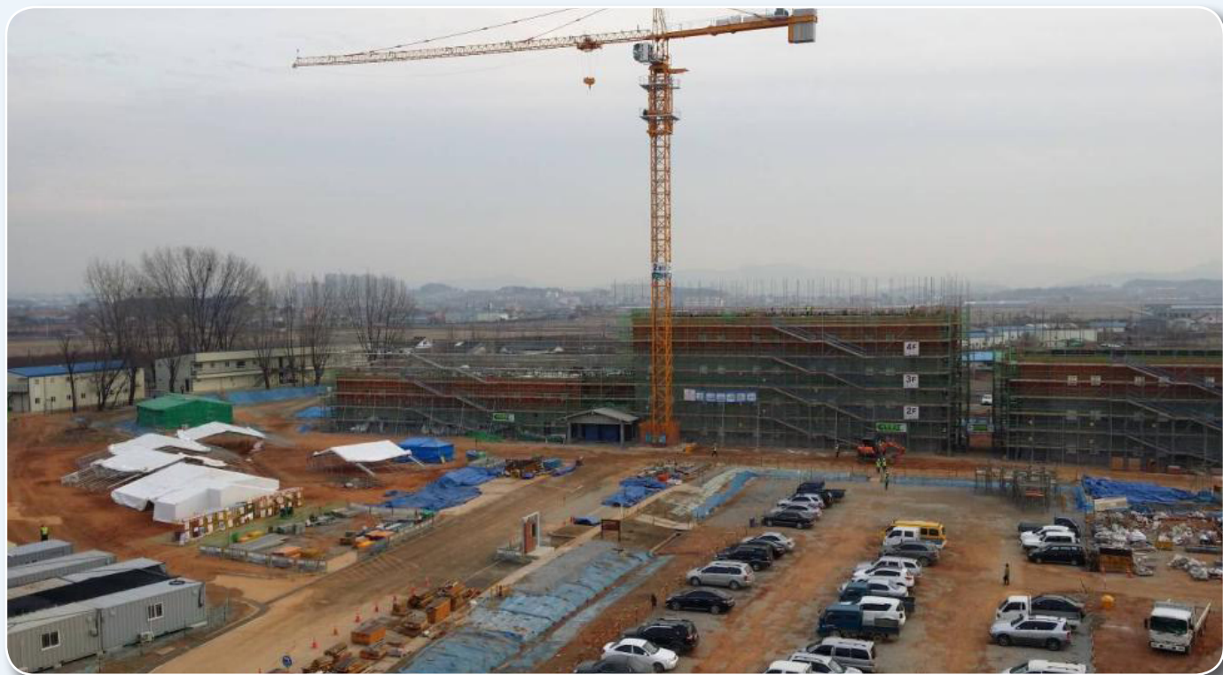
CY08 YRP Hospital Barracks
