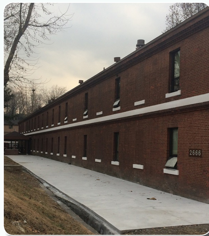
Concrete pad, Building 2666
