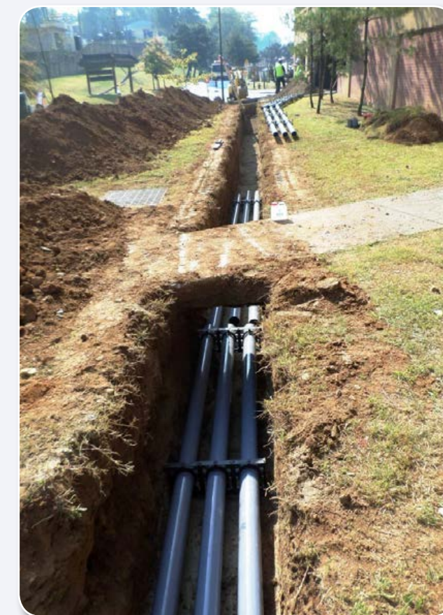
JOC Communication Lines
