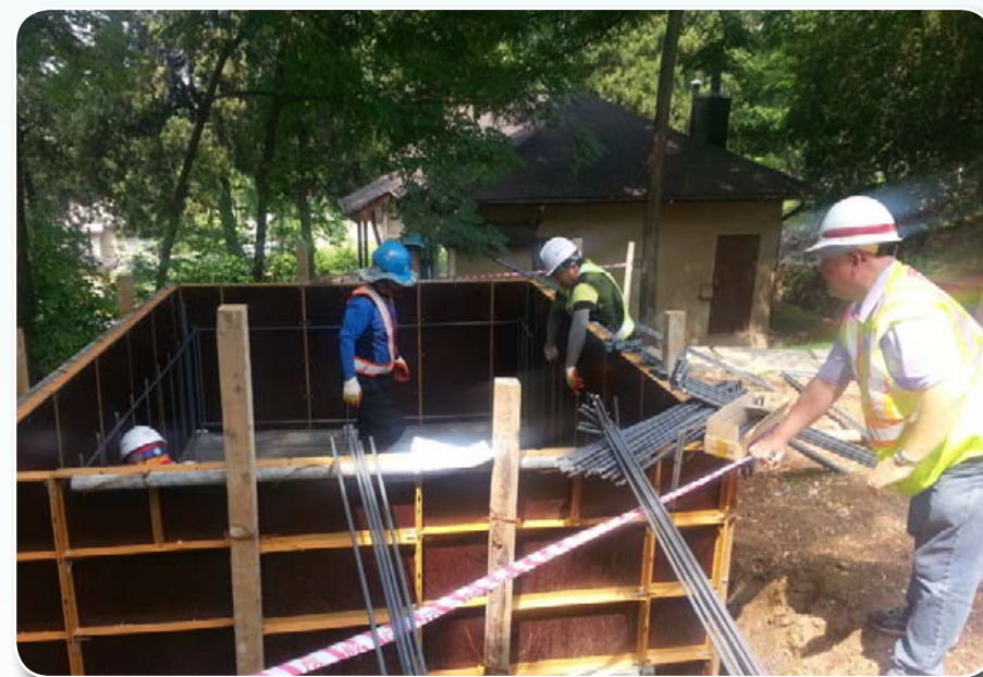
Removal of USTs and Installation of ASTs
