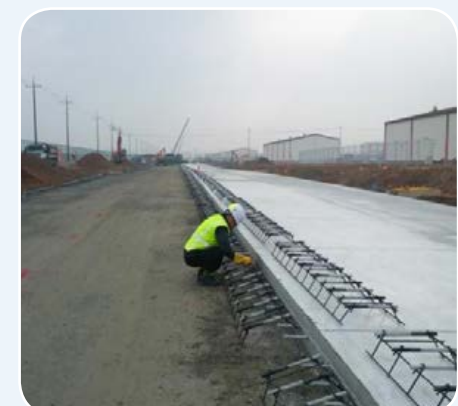
Concrete pavement on A Avenue
