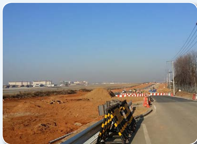
New alignment shift along Airfield Road – old to new
