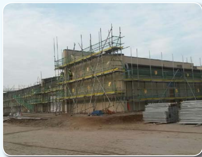
CY13 ROKFC-in-Kind, Convention Munitions Maintenance Facility
