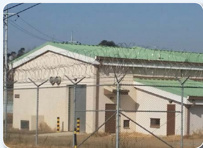
Turned over Chlorination Building to DPW
