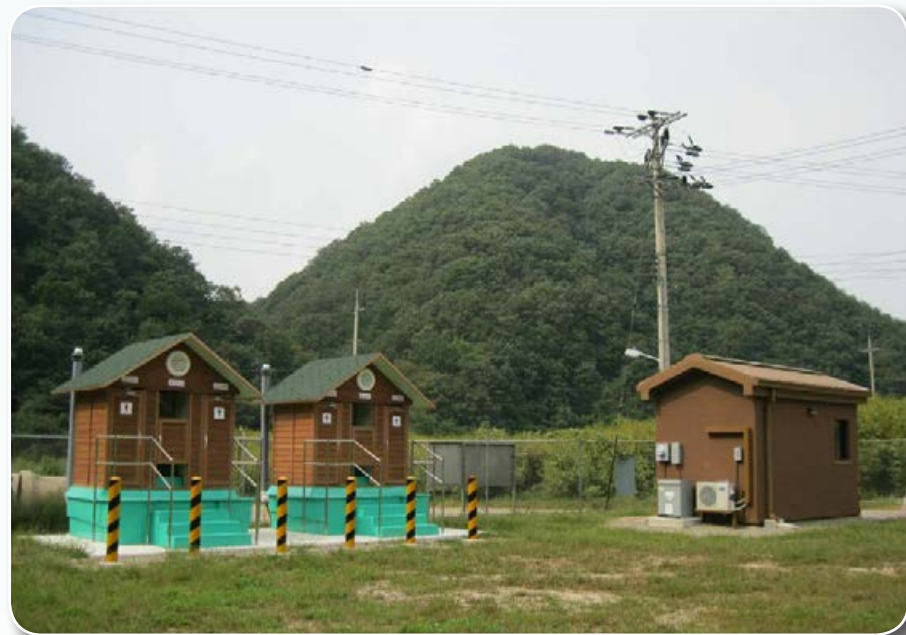
Guard Shack and Composting Toilet, Cherokee Valley, Rodriguez Live Fire Complex
