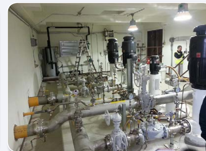
Type IV Hydrant Fuel System
