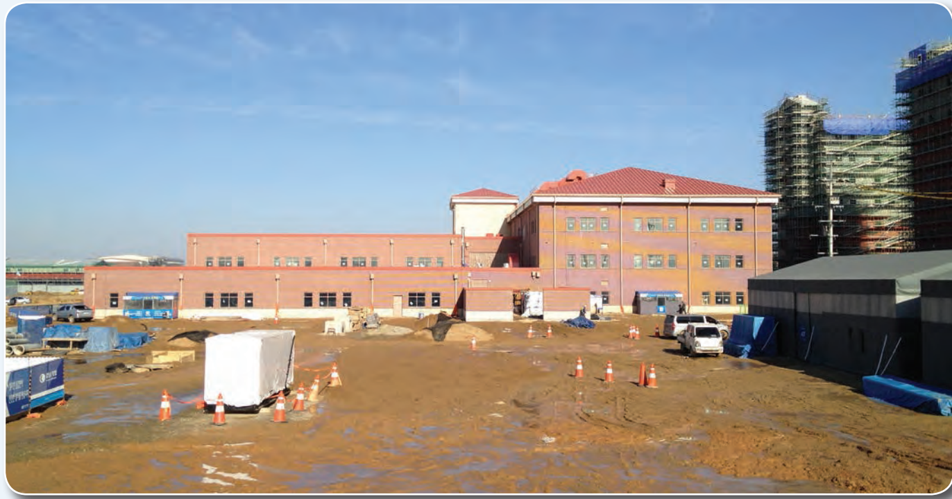
CY10 HBCT Consolidated Headquarters
