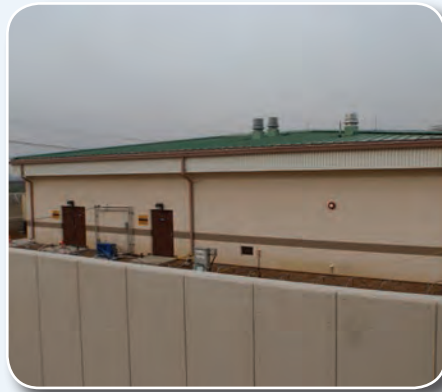
ADN building 93 percent completion
