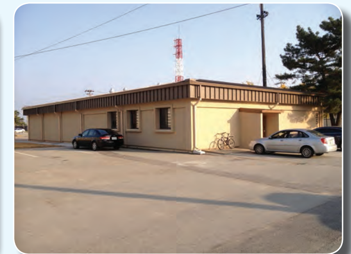
Demolition/Consolidation of B950/954
