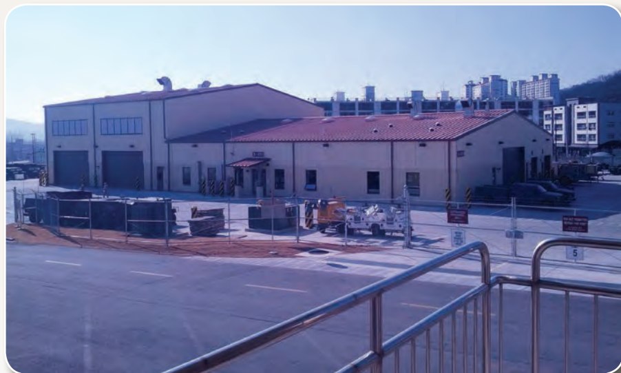
Barracks and Tactical Equipment Maintenance Facility, Camp Carroll
