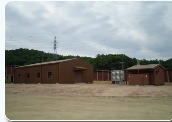
New Facility, Warrior Valley Range
