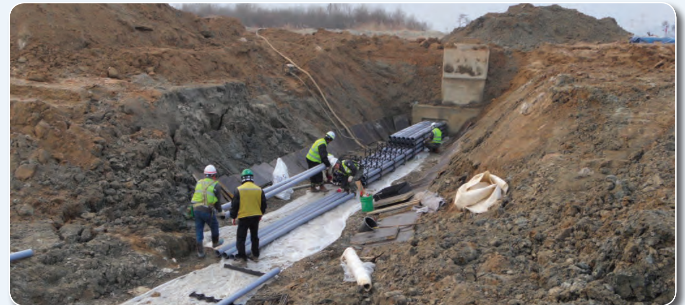
Constructing C4I duct bank
