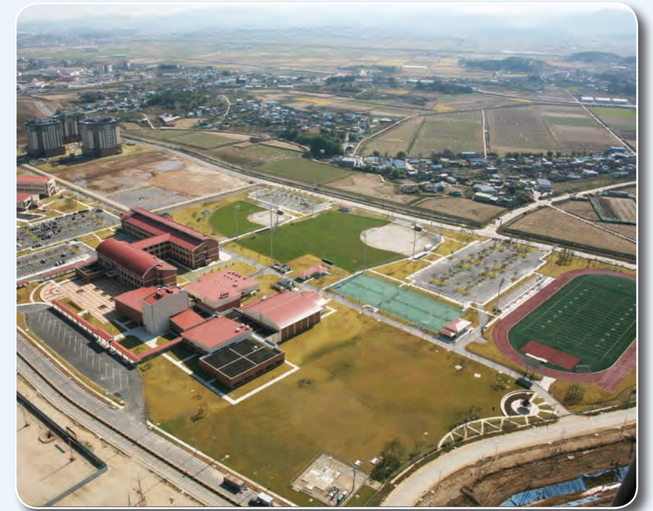
Area view of High School (near) and Elementary School (left)
