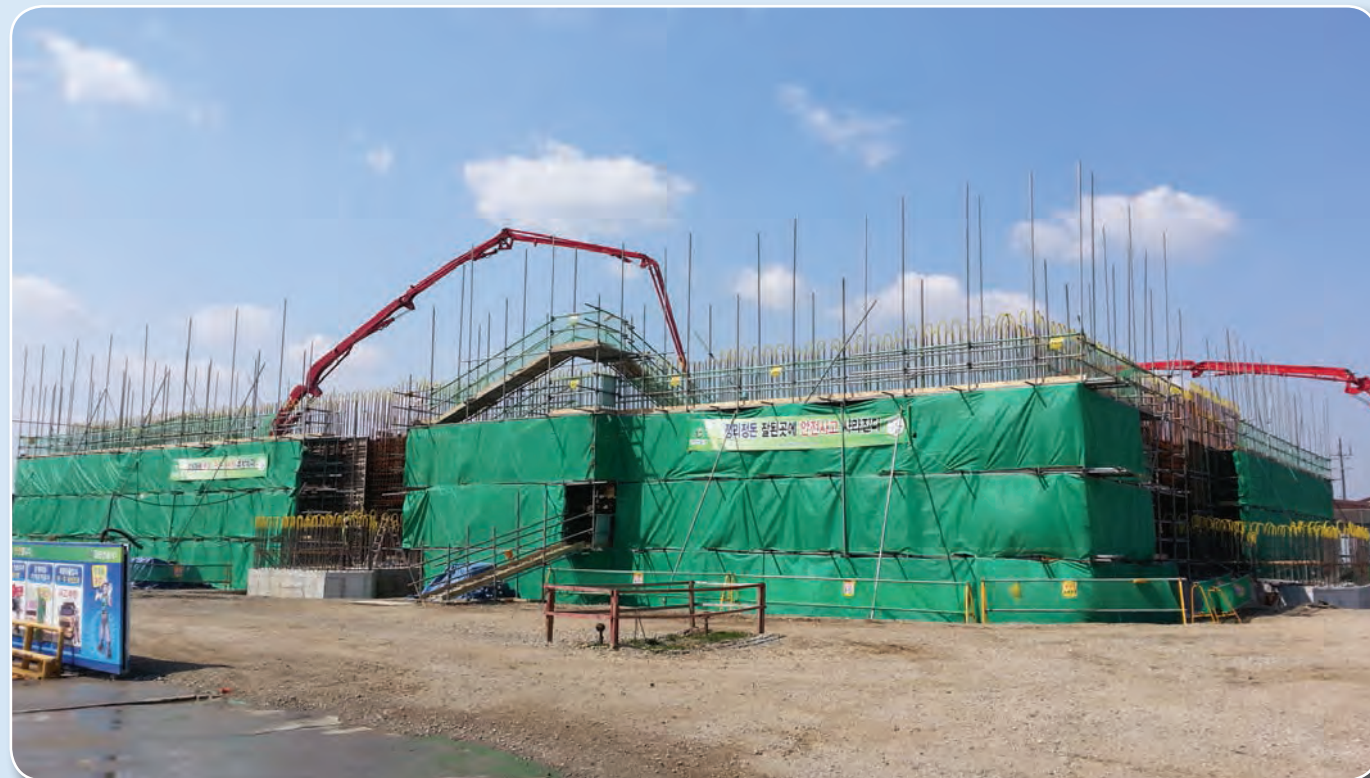
36th Fighter Squadron Operations/Aircraft Maintenance Unit Second floor concrete placement
