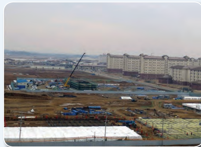
Aerial view of NCO Academy and Transient UPH
