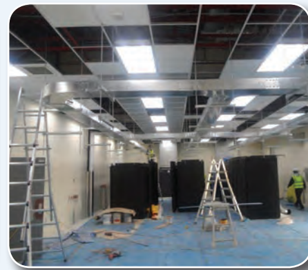
Server room under construction
