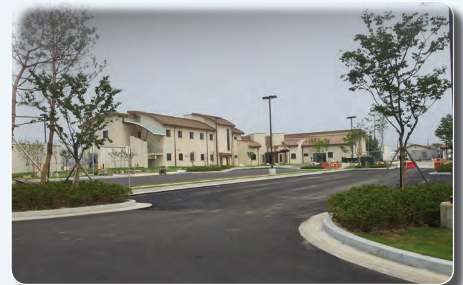
Airfield operations building
