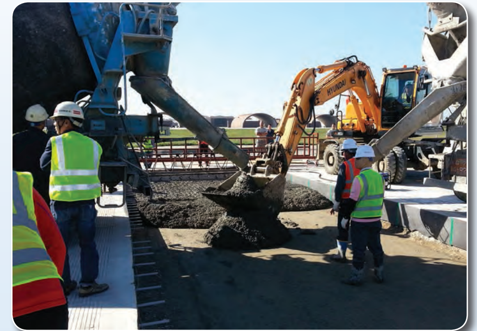
Repair of main runway
