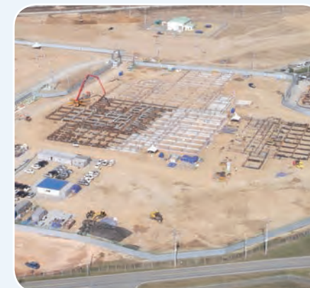
CY08 YRP Eighth Army/CNRK Headquarters – Concrete beams
