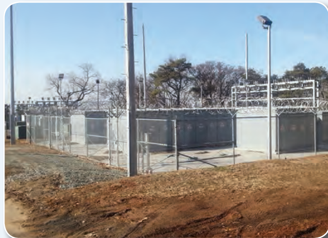
New switchgear at Beacon Hill
