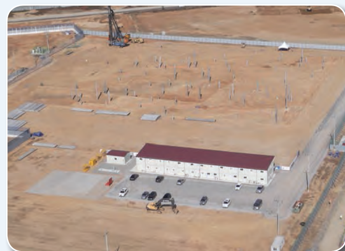
U.S. Korea Command Headquarters – Pile driving
