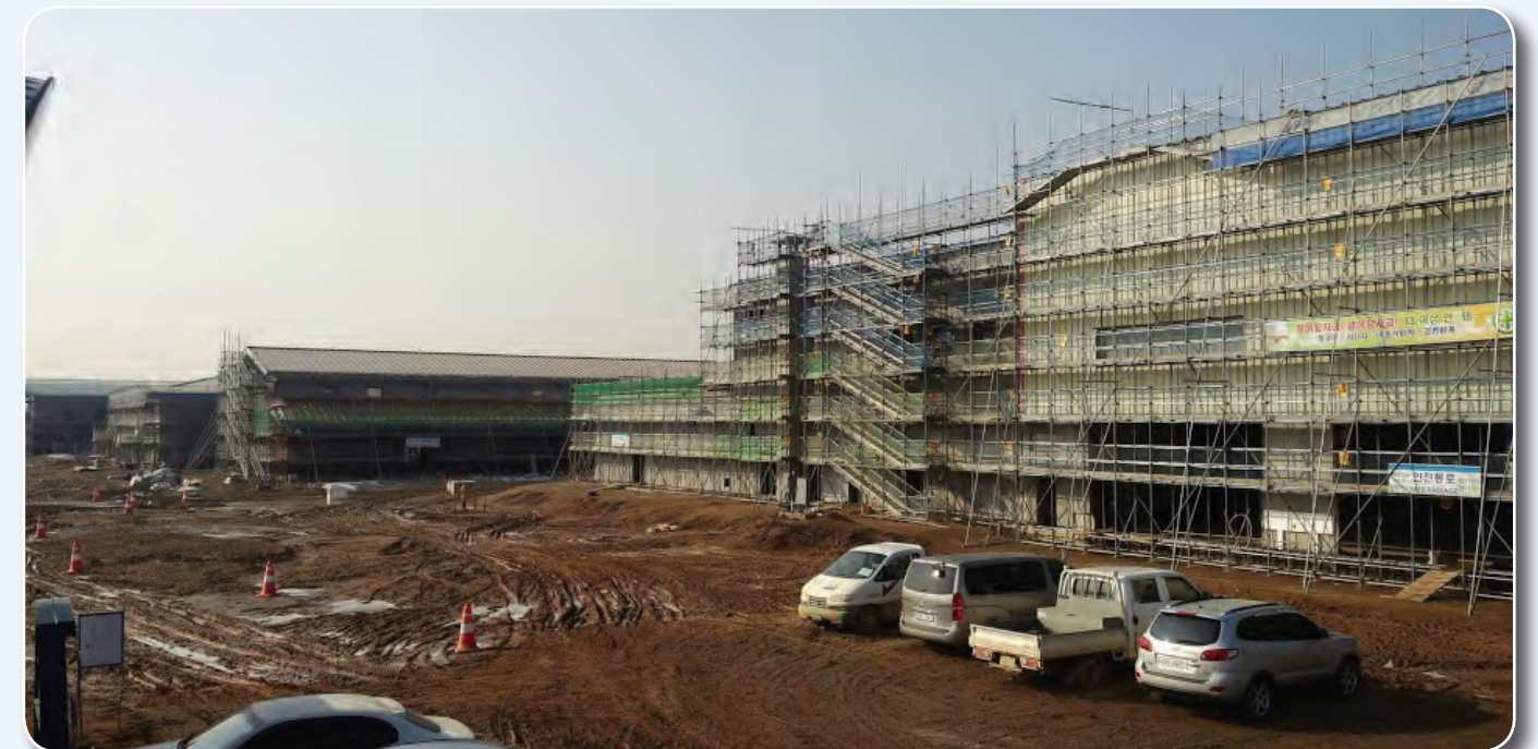
CY11 HBCT Vehicle Maintenance Facility I
