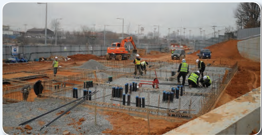
Foundation work for downtown area distribution node in the existing Humphreys
