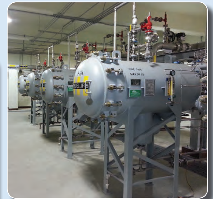
Hydrant Fuel System, Filter building
