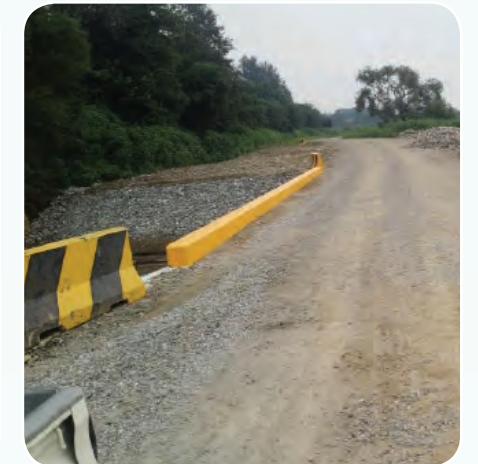
Repair and Upgrade of Maneuver Trail #1, Dagmar-North
