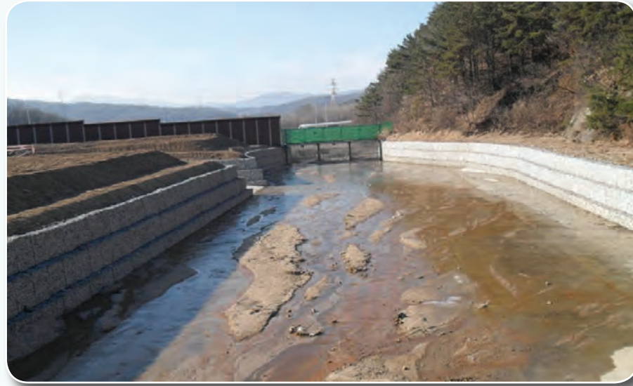
Drainage, Warrior Valley Range
