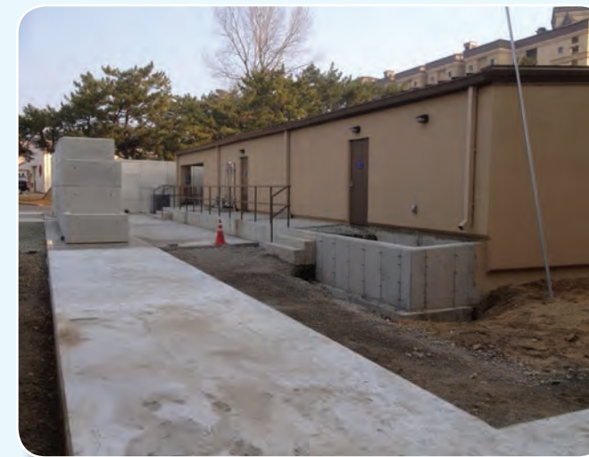
Demolition/Consolidation of B511/512
