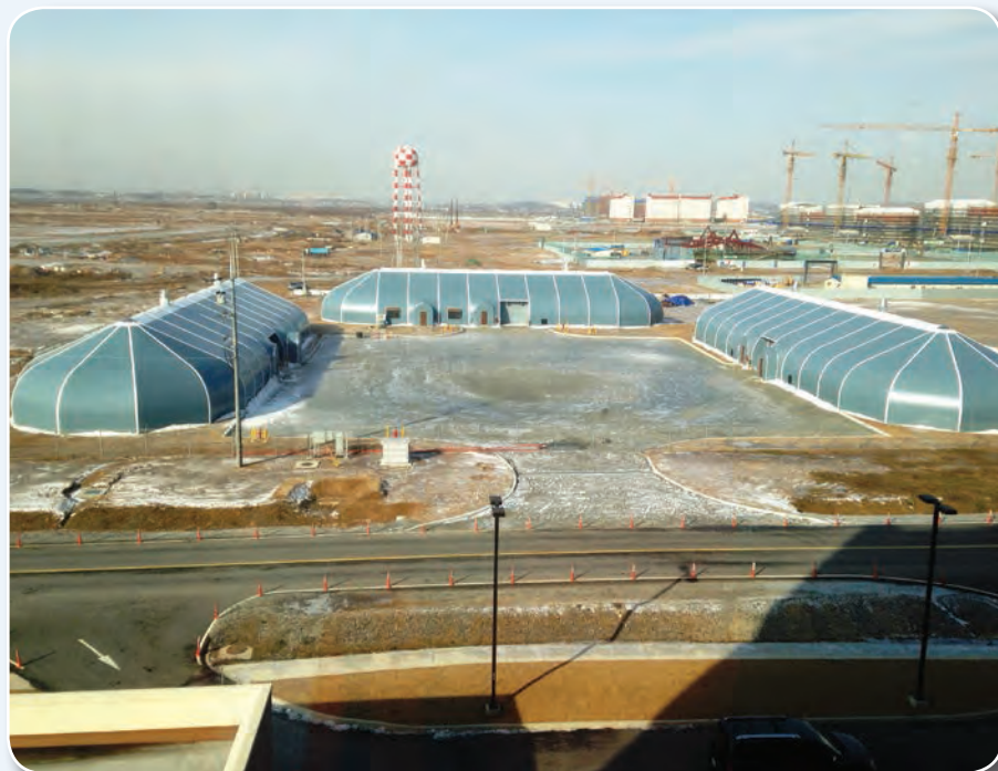
Televideo Center and Swing Space
