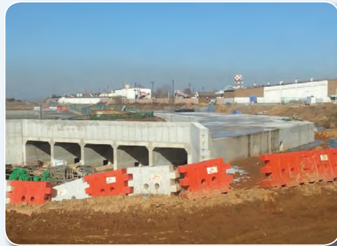
New box culvert next to Alaska Mining Company restaurant in the existing Humphreys
