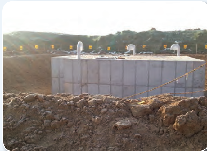
Lift station #18 in the new land (Parcel 2A)
