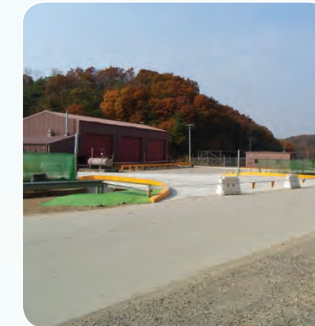
Repair and Upgrade of Tank Trail #1, Rodriguez Live Fire Complex
