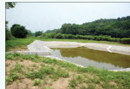
Sediment Basin 3, Story Live Fire
