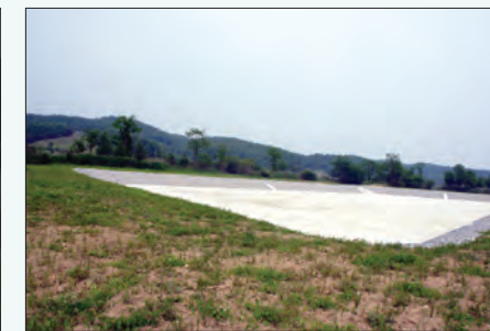
Sediment Basin 4, Story Live Fire
