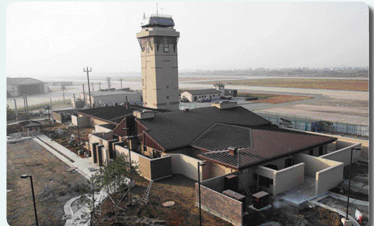
Consolidated Radar Approach Control/Airfield Management Tower Facility
