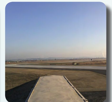
Completed Hot Cargo Pad
