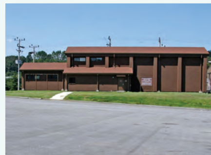
Gym renovation, Warrior Base
