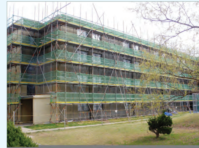
Repair for Dormitory Building 1403
