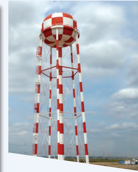
250,000-gallon elevated water storage tank, Parcel 2A
