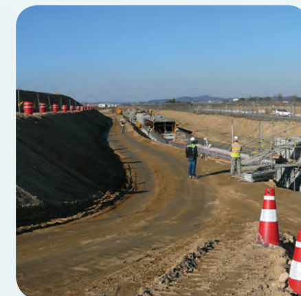
Hot Cargo Pad Under Construction
