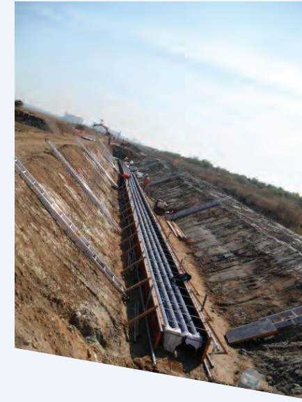
Installation of concrete forms for electric duct bank, Parcel 2B2
