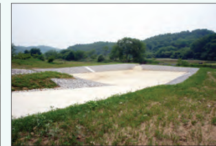
Sediment Basin 2, Story Live Fire
