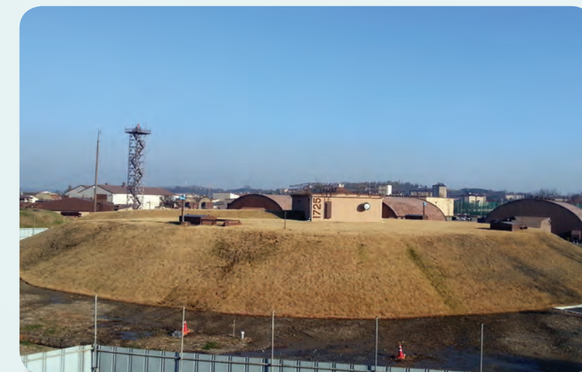
Hydrant Fuel System
