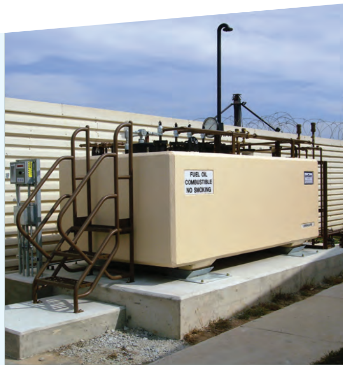
Petroleum, Oil and Lubricants Storage Tank System
