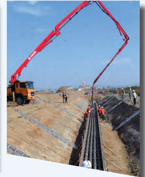
Concrete placement for electric duct bank, Parcel 2B2
