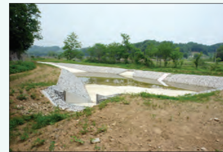
Sediment Basin 1, Story Live Fire
