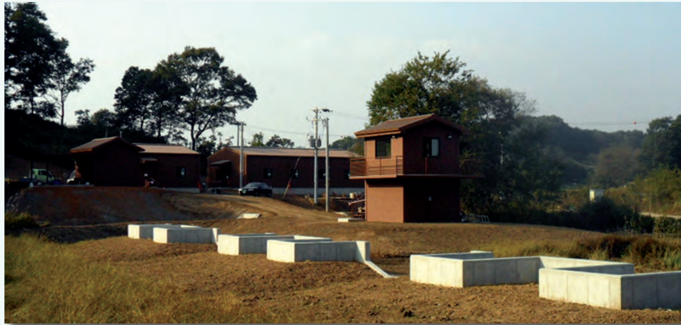
Range Operations Control Area, Story Live Fire Complex
