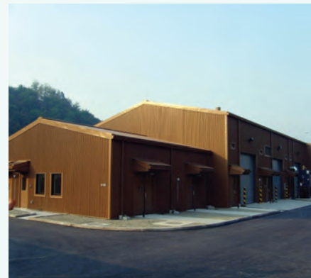
DPW Sub-station, Yongpyong
