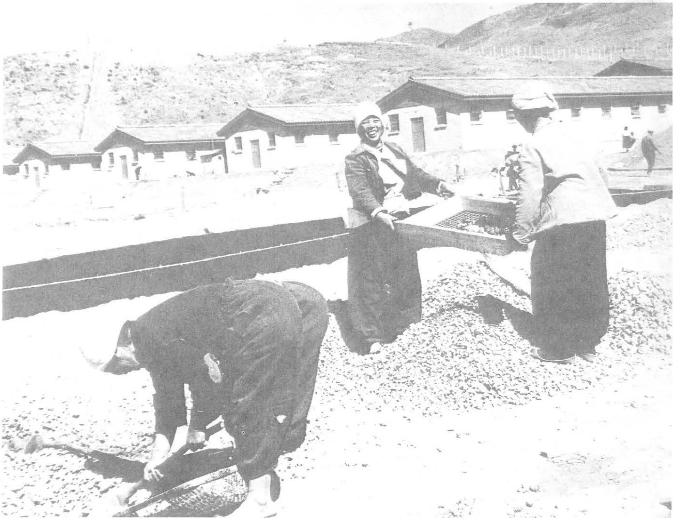
Laborers screening aggregate for road construction, Camp Ames. New enlisted barracks in background.
