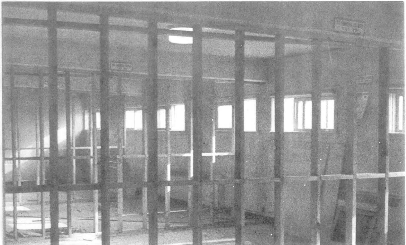
MVA modernization of superhooch
