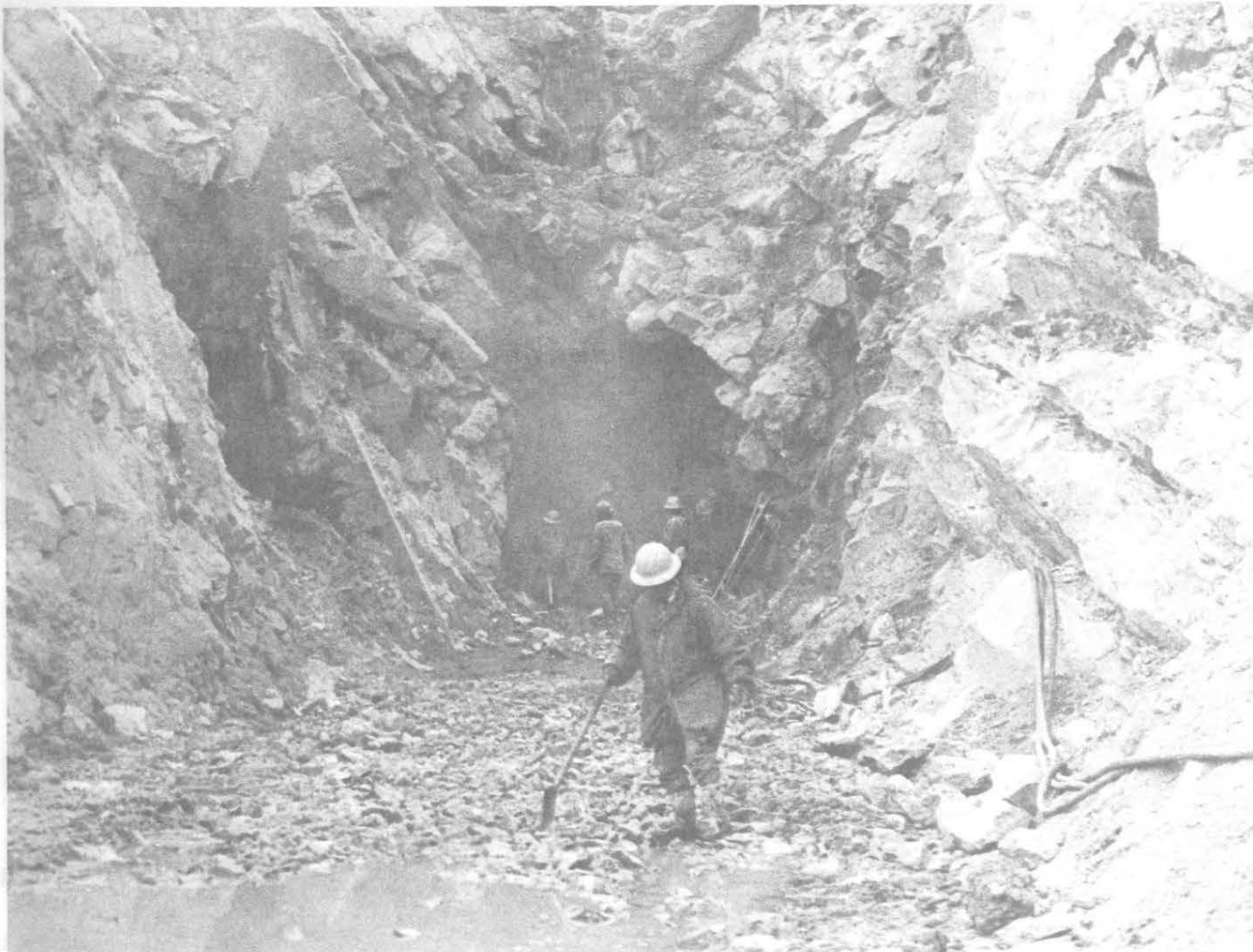
Tunnel excavation, Tango
