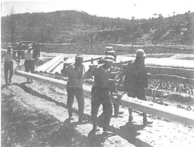
Laborers transporting the easily damaged pipe
