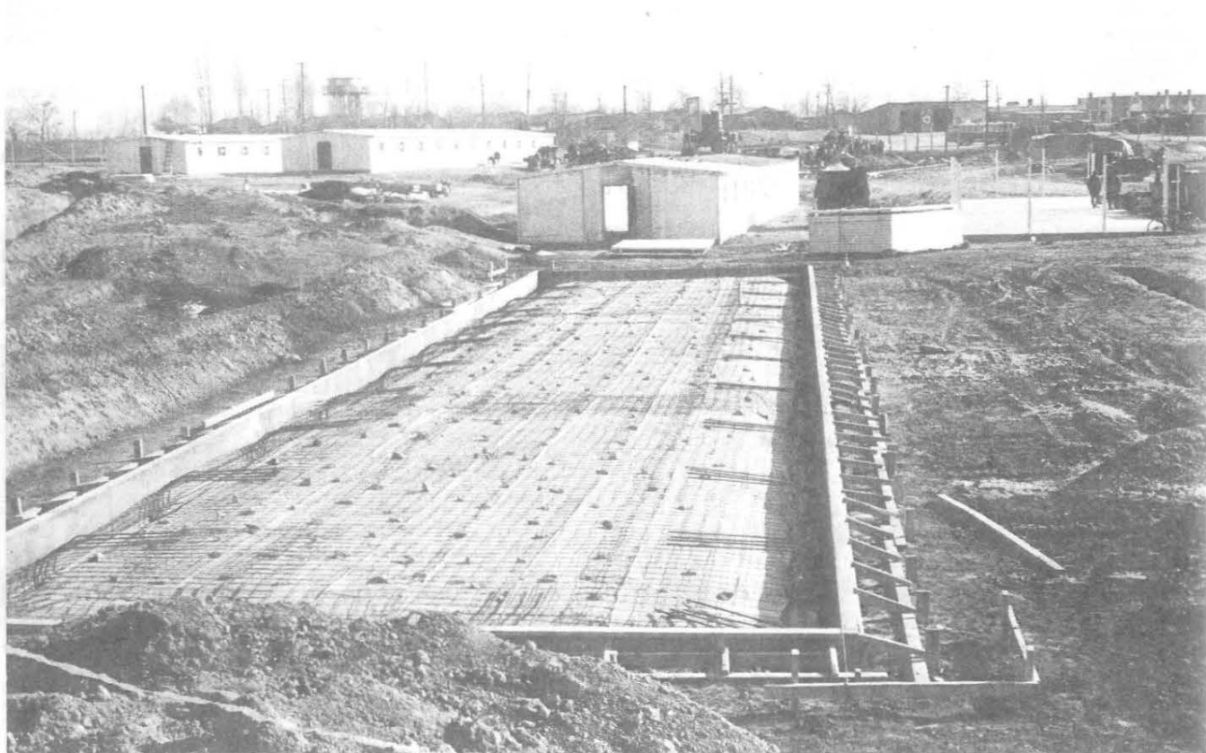
Engineer troop construction segment of housing project at Camp Humphreys
