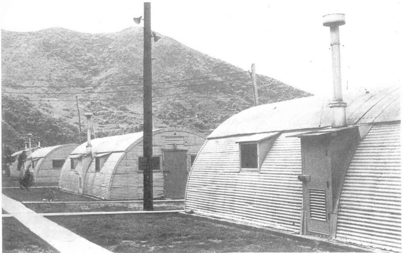
Warm air furnaces installed within quonsets, NCO Academy
