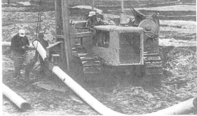
Bending coated pipe to conform with variations in the course of the pipeline
