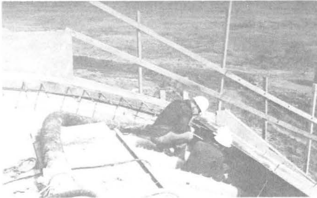
Placing concrete on first aircraft shelter, Osan Air Base
