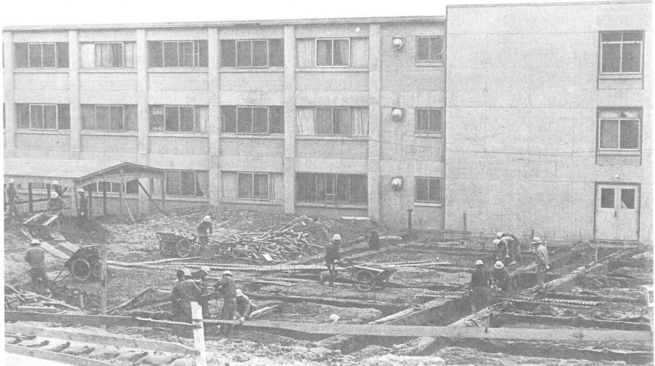
Initial stages of building one of three units to connect and expand two extant barracks, Camp Carroll
