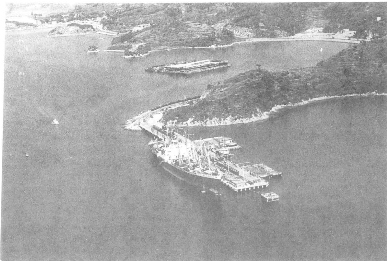
View of Chinhae complex in 1975. The road and railroad tracks can be seen arching to the right past some of the support facilities and then on to left background.
