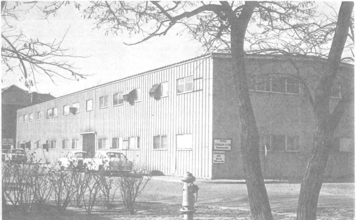
Pre-engineered office building, FED Compound, Seoul
