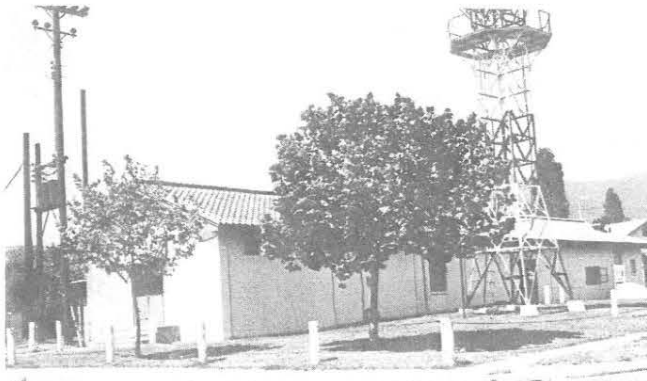
Telephone exchange, Hialeah Compound, Pusan, in 1975, microwave equipment is a recent addition
