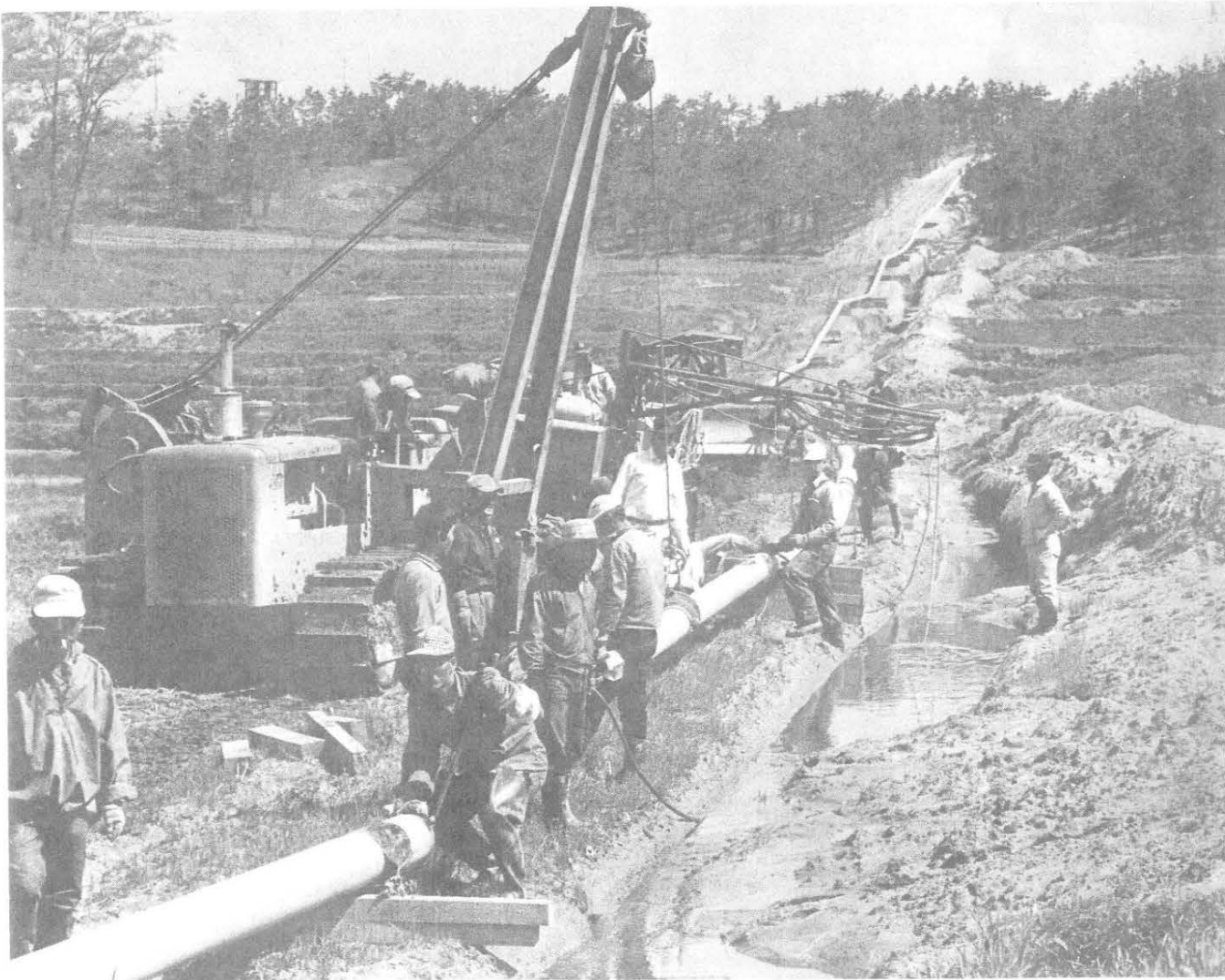
Laying of pipe for trans-Korea POL pipeline
