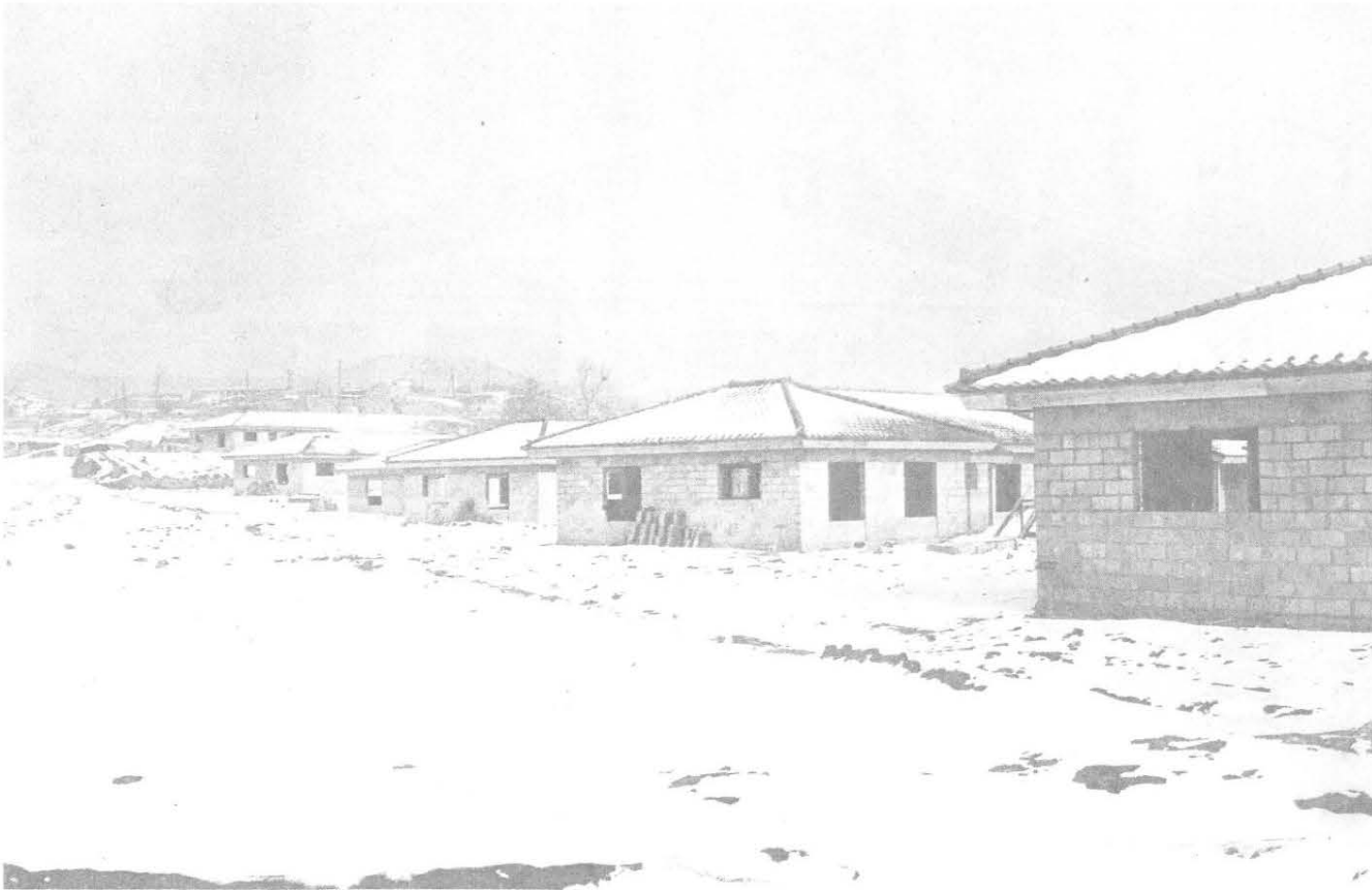
Family housing under construction for the Office of the Economic Coordinator, Seoul. The units consist of locally-procured roof tiles and concrete blocks.
