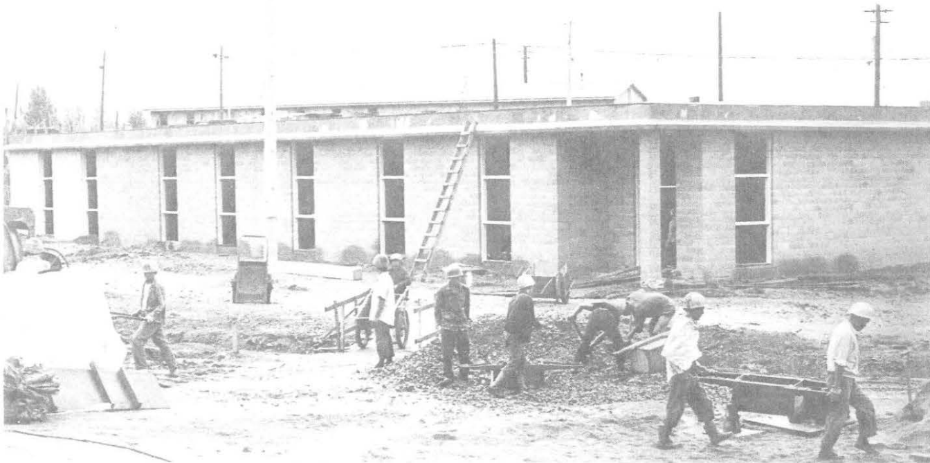
500 man mess hall project, Camp Red Cloud
