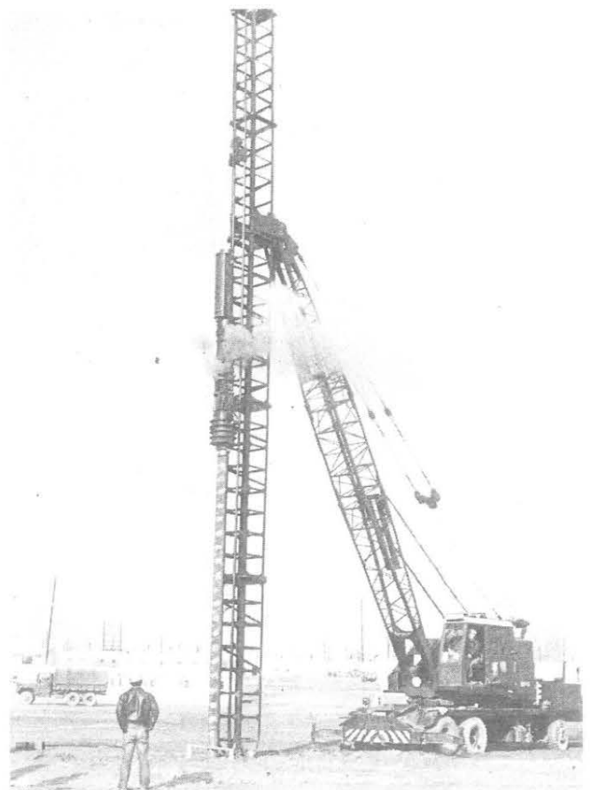
Pile driving for one of the barracks foundations, Camp Humphreys
