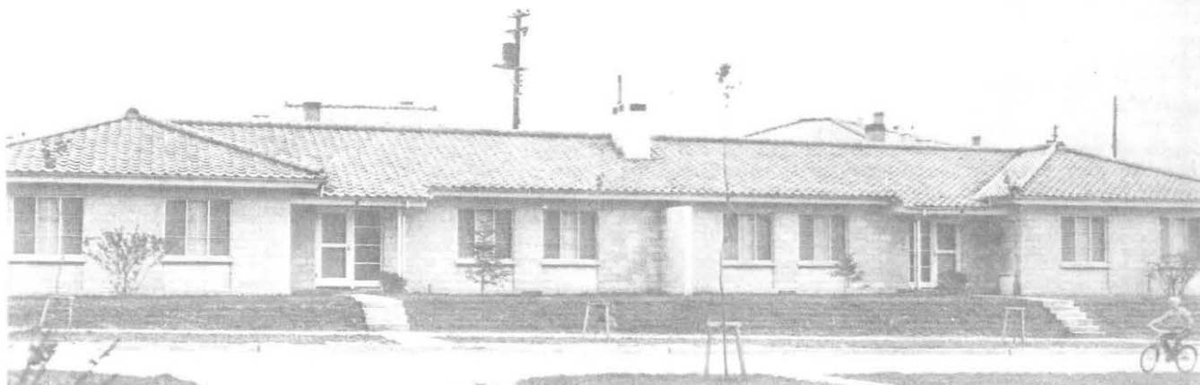
Three bedroom duplex built for PROV-MAAG-K, Seoul
