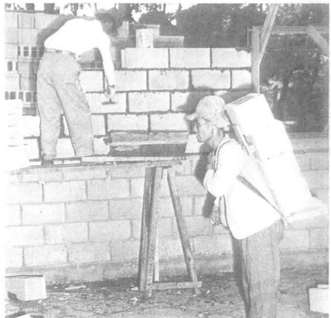
Worker hauling concrete blocks on a back pack for 6-man BOQ Seoul
