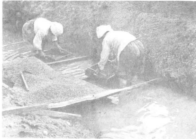
Workers hand washing aggregate
