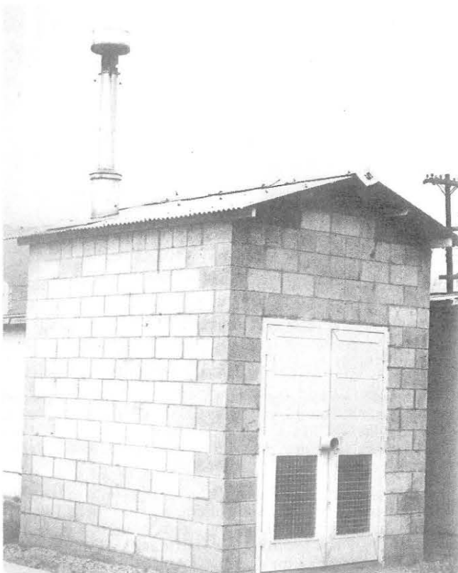
Warm air furnace housed separately, NCO Academy, Camp Casey
