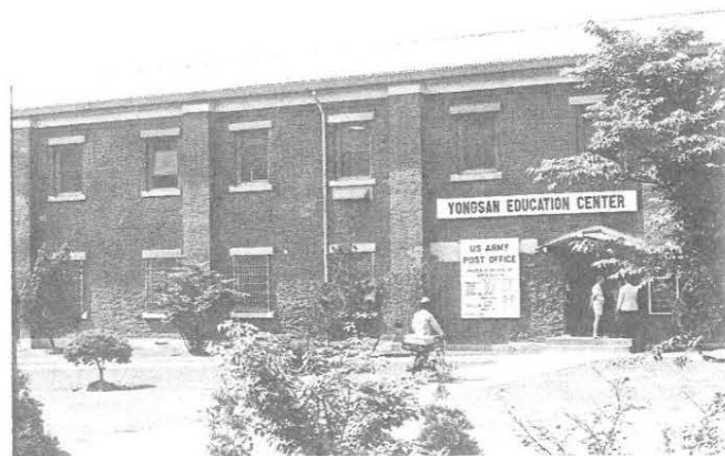
Building 2212 after restoration, Seoul
