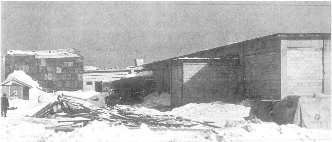
Partially complete commissary addition, Wakkanai, with winterized portion on the left
