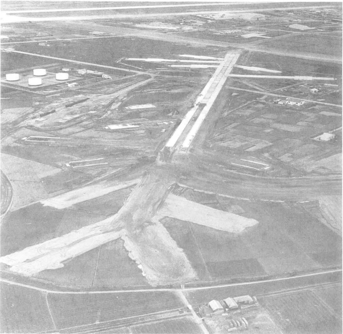
Partial completion of dispersal pads and associated paving, Kunsan
