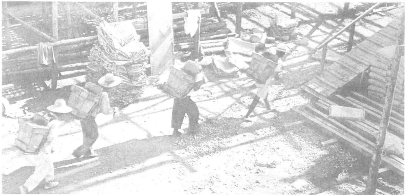
Transporting material by pack-box
