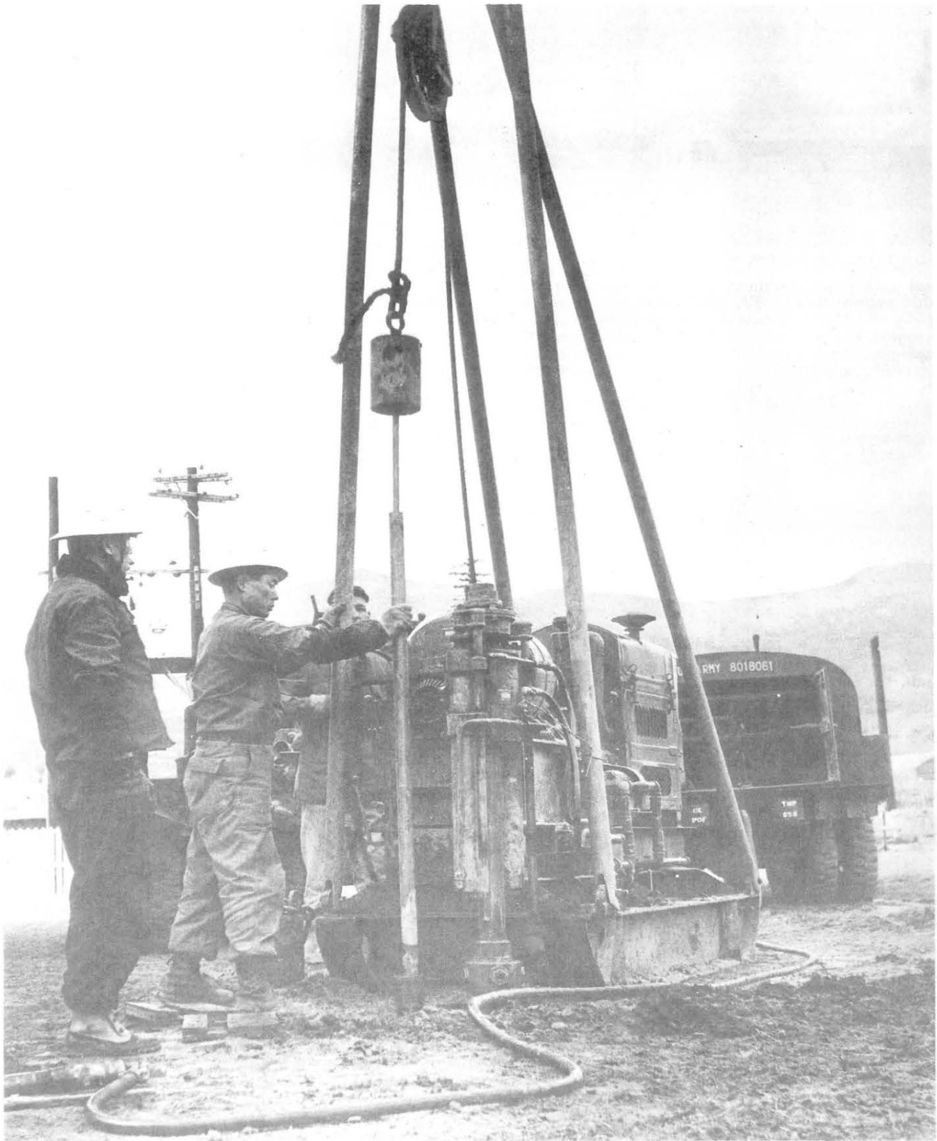
FED employee inserting core rod prior to taking sample for moisture content, Hialeah Compound, Pusan
