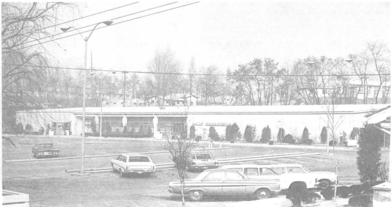
1975 view of Main Exchange
