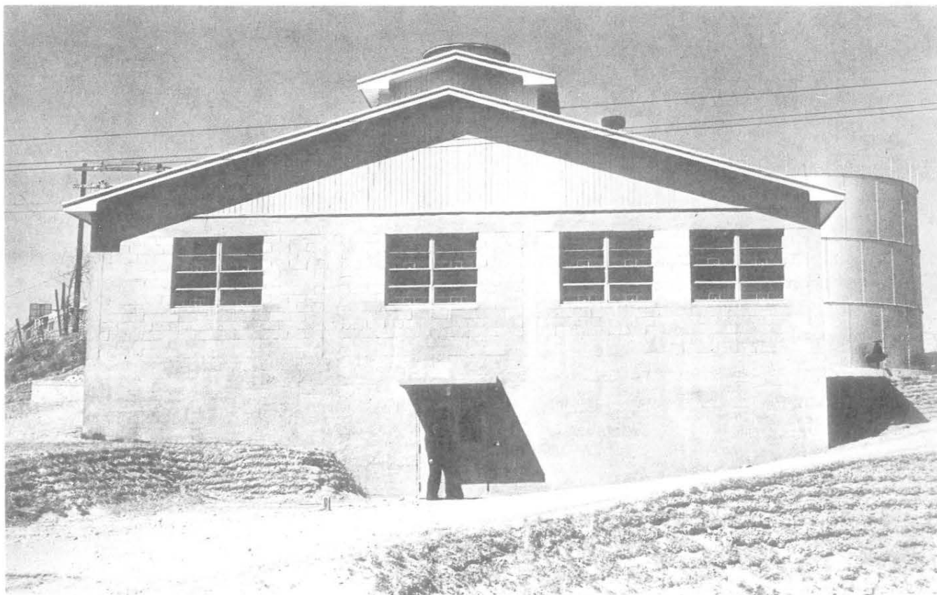
Water treatment plant, Osan Air Base
