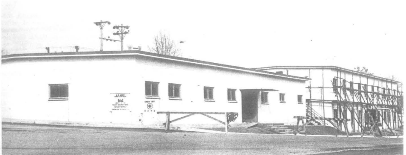
Almost finished community facility, Camp Humphreys
