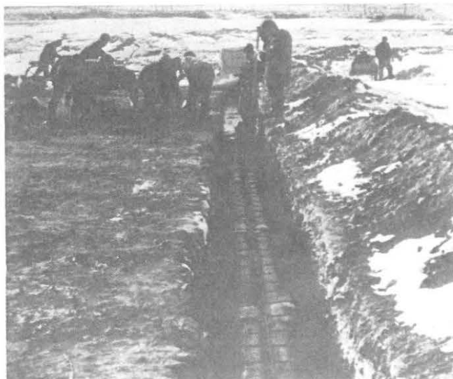
Laying conduits across runway, Yang-gu, ALOC Airfield
