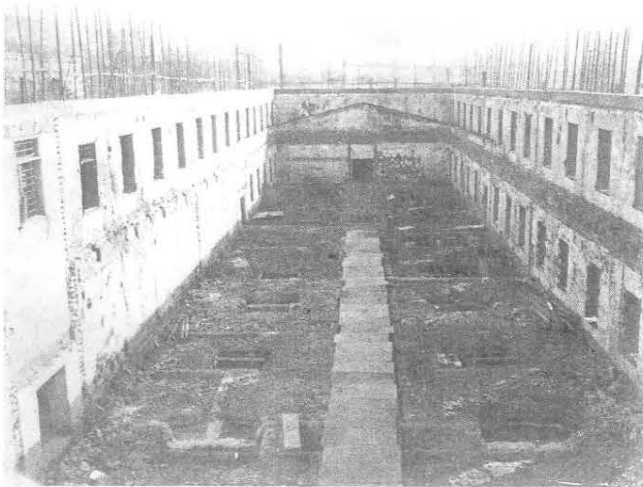
Fire-gutted Building 2212, Seoul
