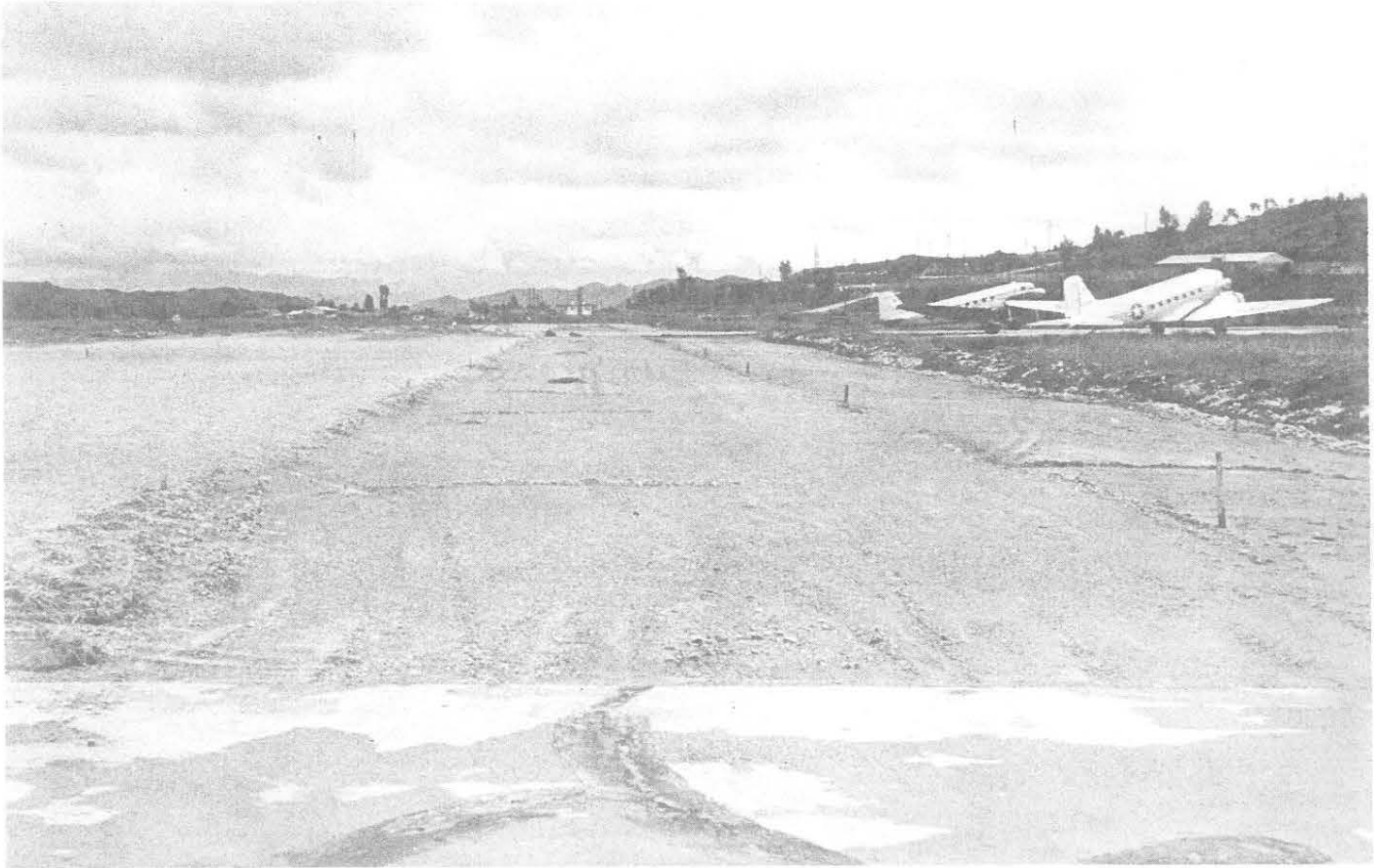
Taxiway improvement, Osan Air Base
