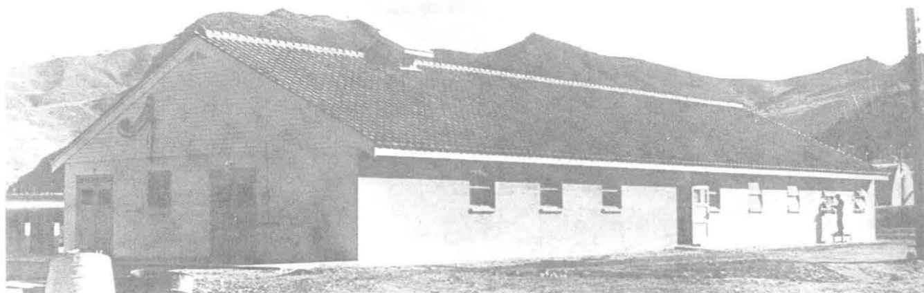
Nearly completed augmented Company size mess hall, Mortar Battery area, 1st Cavalry Division
