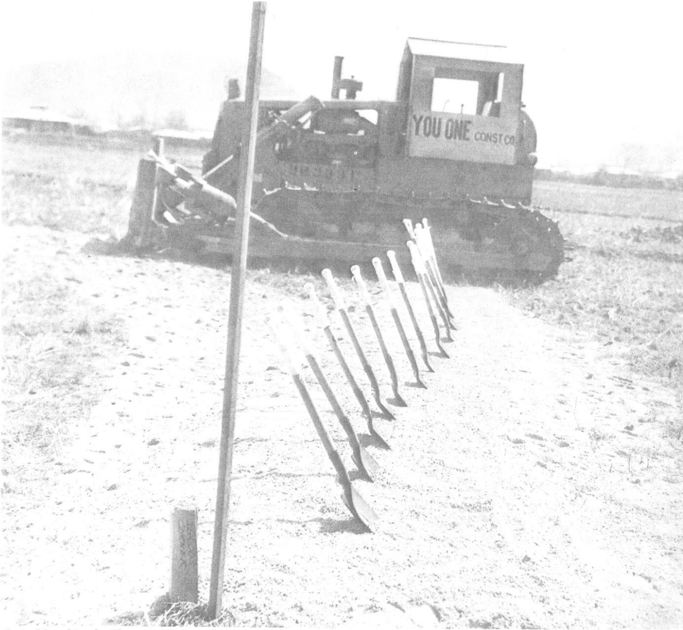
Ground breaking for Kwangju Air Base ordnance storage facility
