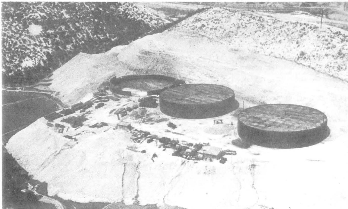
Three fuel storage tanks under construction, Pohang
