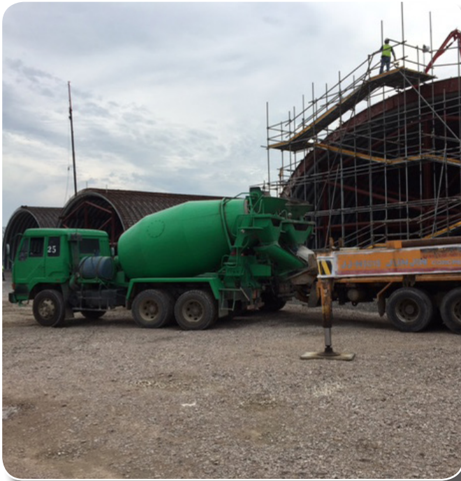
Far East District Kunsan resident office engineers inspected concrete placement of a hardened aircraft flow through shelter Aug. 1. Concrete placement for this project requires 110 trucks of concrete which takes around 18-20 hours. A total of 10 shelters will be constructed at Kunsan Air Base. (FED file photos)
