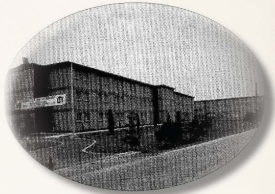
Unaccompanied enlisted personnel housing units at Kunsan Air Base opened in October 1985.
