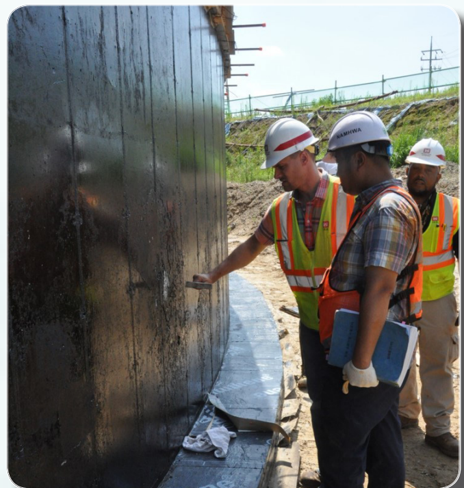
(Above) Nick Dubas (POL-MCX structural engineer, left) revealing concrete delamination to contractor (middle) and Tim Colón (FED, right) at Camp Humphreys. (Photo by G. Etter)
