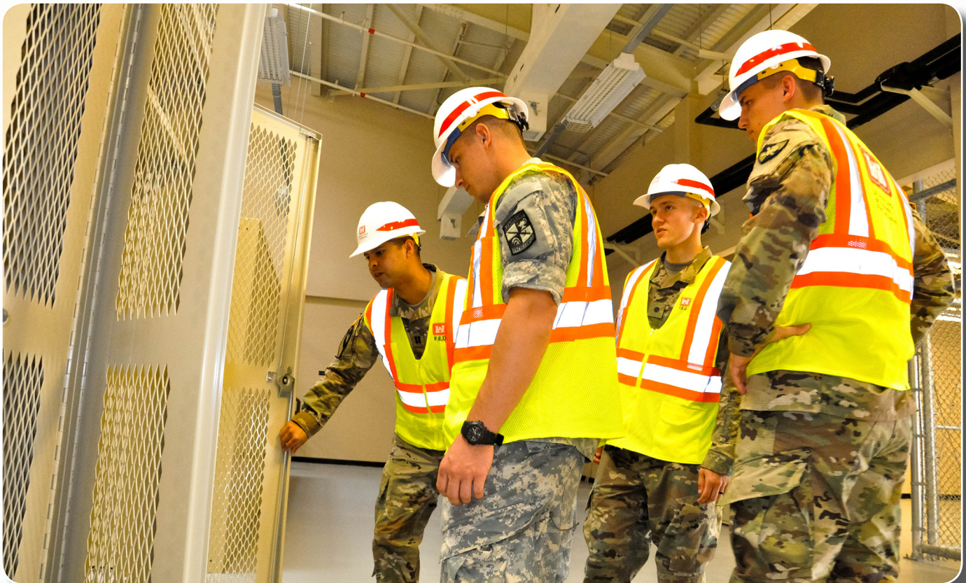
Capt. Rodolfo Martinez (far left) a project engineer, inspects a wall locker and explains deficiencies to Cadet Drako Gagnon (left) University of Wisconsin-River Falls, Cadet Tim Gephart (center) United States Military Academy, and Cadet Caleb Kowalski University of Wisconsin-Madison, during a site walk on July 27, 2017. (Photo by Antwaun Parrish)
