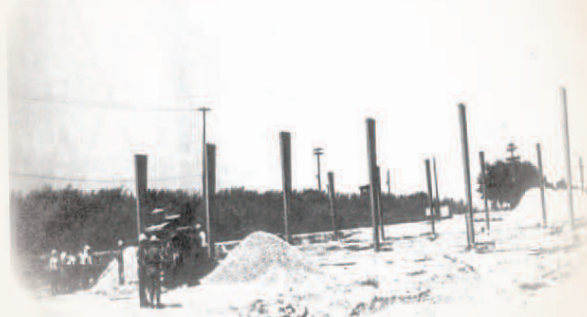
Engineer troop project, ASA hangar, Humphreys, in August 1975
