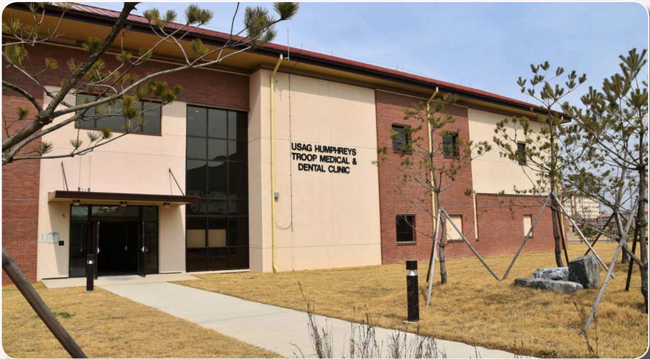
The U.S. Army Garrison Humphreys MEDS 50 Troop Medical and Dental Clinic was transferred and signed as real property to USAG Humphreys Department of Public Works, effective March 24. The project was completed thanks to the efforts of the Medical Resident Office. (Photo by Antwaun J. Parrish)
