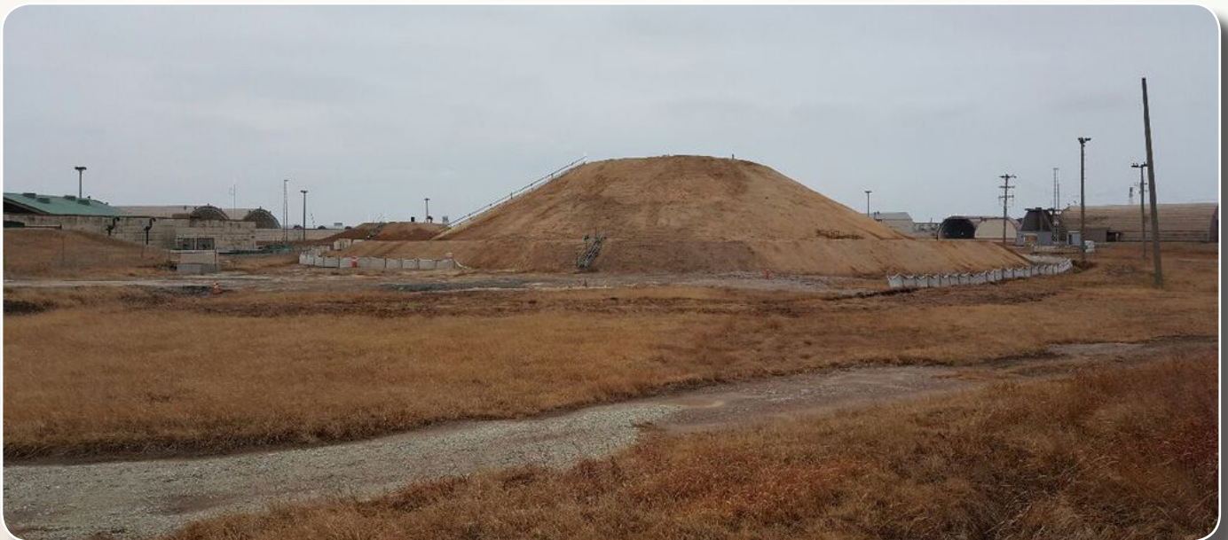
Construction on flow-through shelters at Kunsan Air Base has begun. Kunsan resident office engineers expect the project to be completed by early 2019. (FED file photo)
