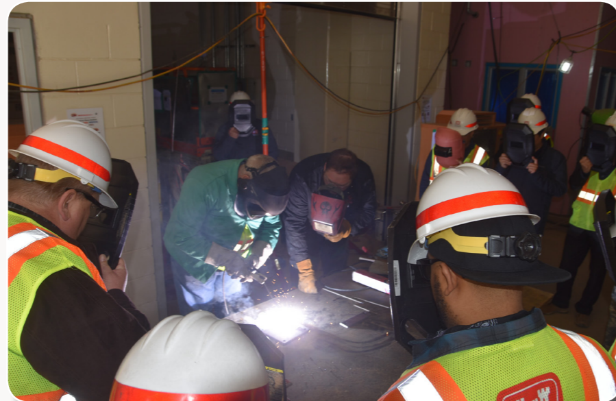
A class participant welds a piece of metal during the U.S. Army Corps of Engineers Far East District quality verification course March 13-17. The course teaches the participant how to interpret the various methods and techniques employed in weldments and assuring the quality of welds. (Photo by Antwaun J. Parrish)
