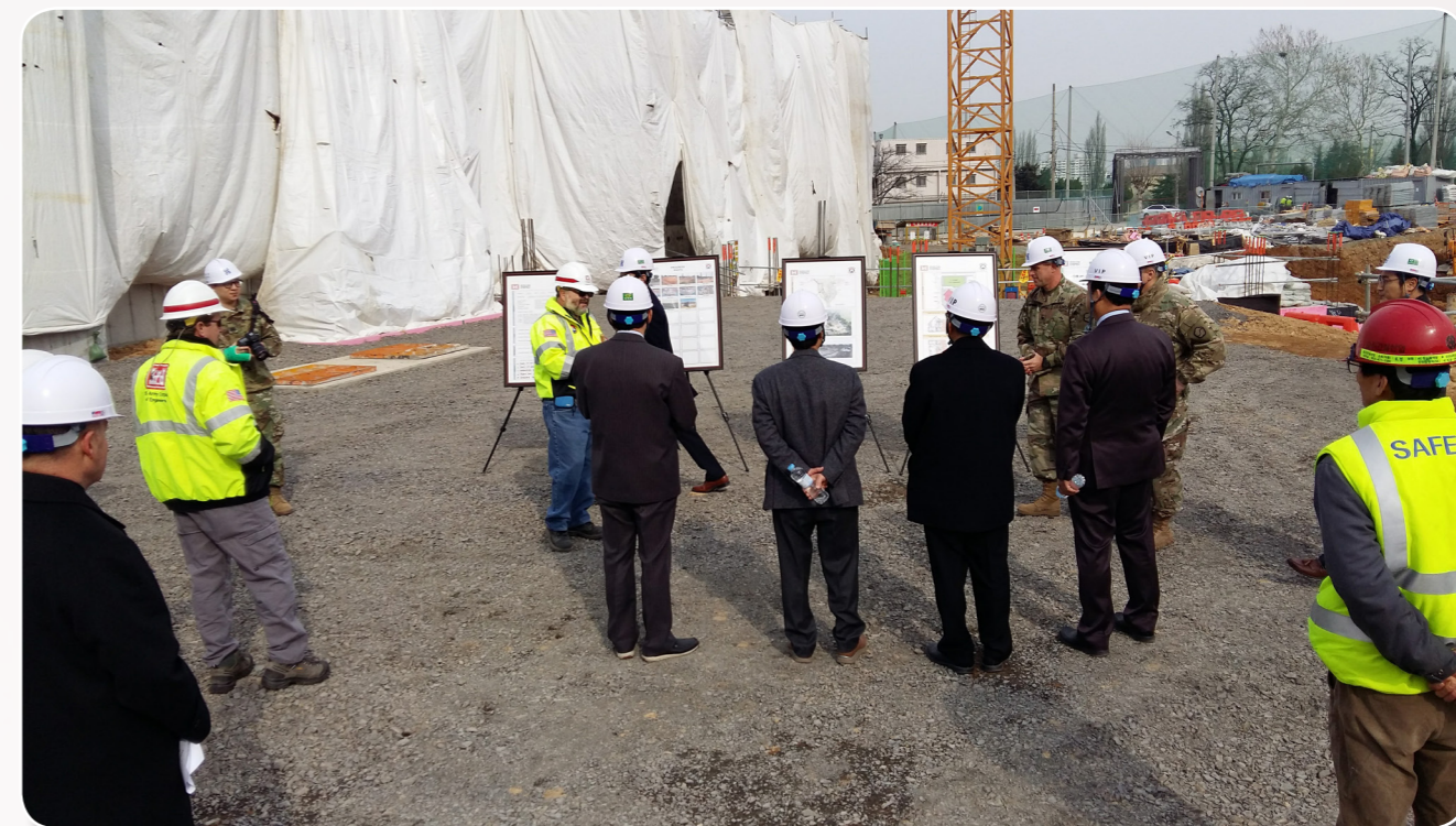
Far East District southern resident office engineers gave briefings on the Daegu middle and high school project and the Army Family Housing Tower project at Camp Carroll to Korean cultural advisors and Daegu high school principal Altorn Grade Feb. 8. (FED file photo)
