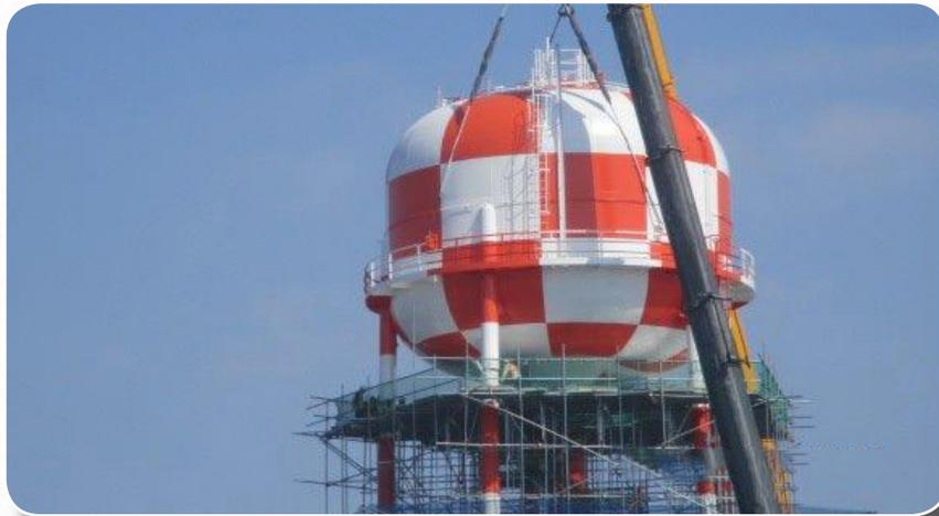
*Far East District Parcel 2 Resident Office recently placed the last of four water towers at U.S. Army Garrison Humphreys. The towers are 50 meters high and can each hold 250,000 gallons of water. These towers will provide a safe and steady supply of water for drinking and fire protection for the army community. (Photos by RT Hodge)*
