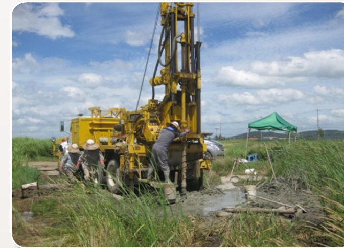
CME-75 Truck-mounted drill rig at Yongsan Relocation Project site at USAG Humphreys. (FED file photo)
