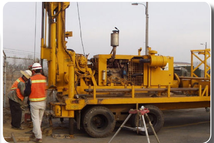
(left) CME-75 Truck-mounted drill rig at Yongsan Relocation Project site at USAG Humphreys. (right) CME-75 Trailer-mounted drill rig at the existing boundary of USAG Humphreys. (FED file photos)
