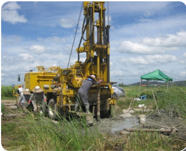
(left) CME-75 Truck-mounted drill rig at Yongsan Relocation Project site at USAG Humphreys. (right) CME-75 Trailer-mounted drill rig at the existing boundary of USAG Humphreys. (FED file photos)
