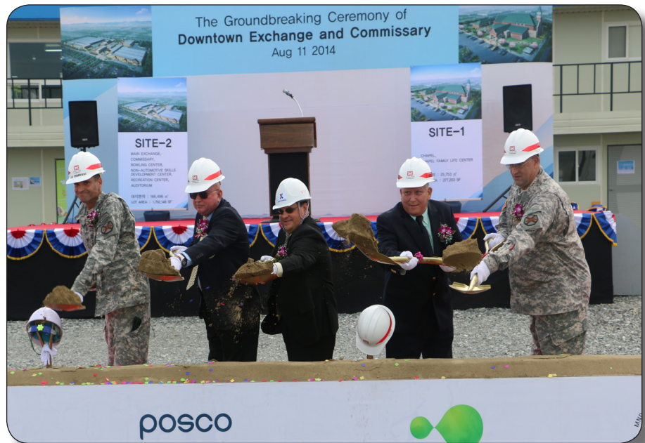
Ground was broken for the new “downtown” area, featuring a new Exchange, commissary and bowling center among other facilities, at U. S. Army Garrison Humphreys, Aug. 11. The project will also see the construction of an auditorium, chapel, chapel family life center, an arts & crafts center, recreation center, plaza and parking. When completed, these facilities will provide retail shopping, groceries, entertainment, recreation and religious services. (U.S. Army photo by Steven Hoover)
