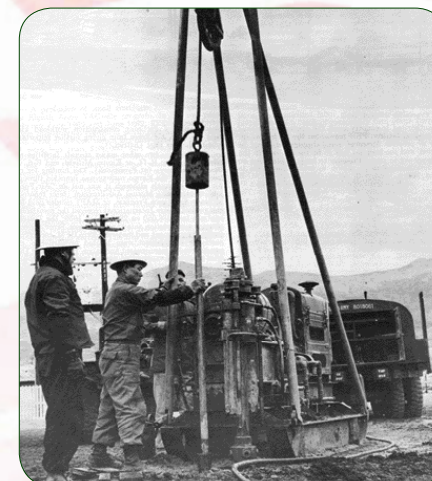
FED employees insert a core rod to take a soil sample at Camp Hialeah, 1960
