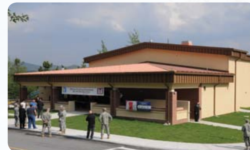
The recently completed multipurpose training facility at Camp Carroll will allow U.S. Army Garrison Daegu to conduct unit training. (Photo by Patrick Bray)
