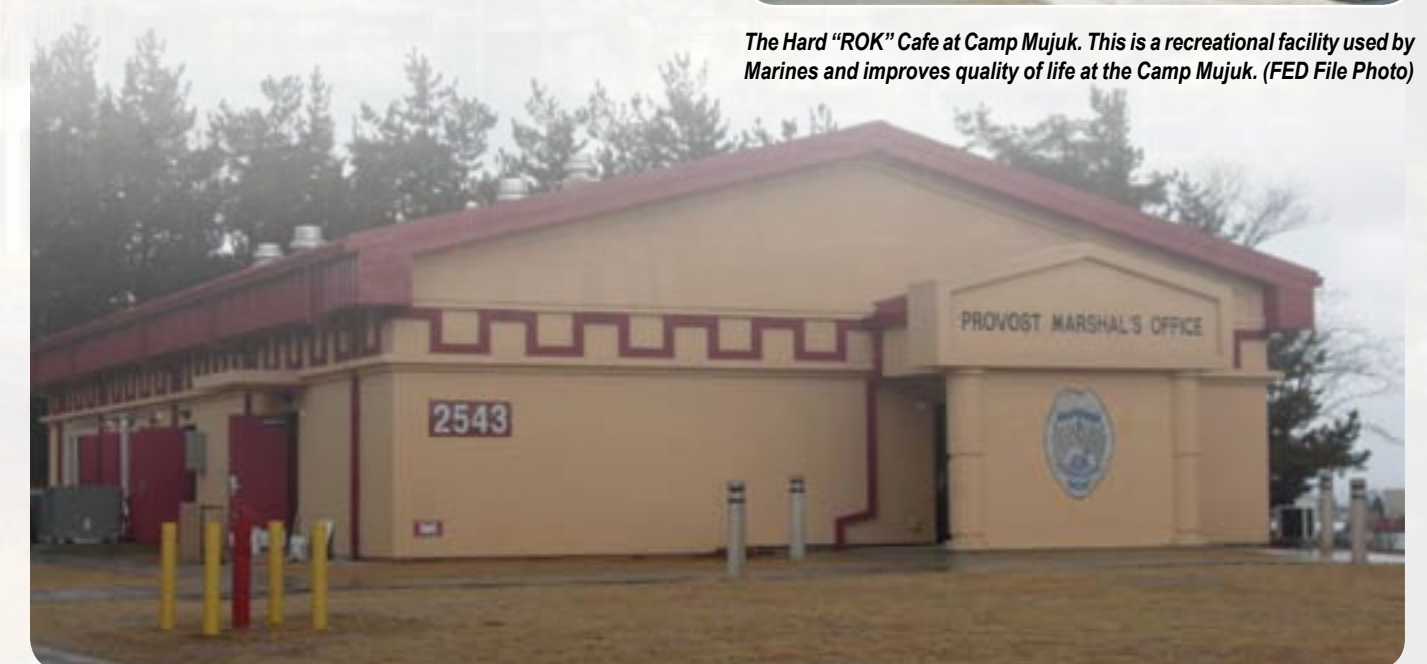
The new provost marshal's office for the U.S. Marine Corps at Camp Mujuk constructed by the U.S. Army Corps of Engineers Far East District. (Photo provided by FED Southern Resident Office)
