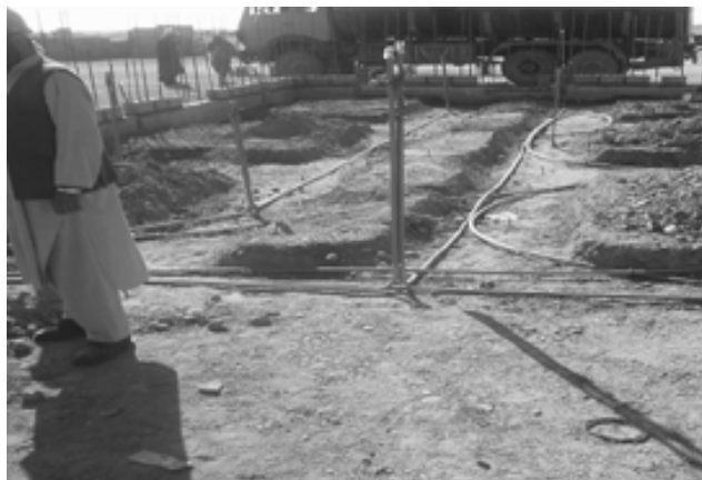
Barracks CMU walls going up and interior electrical stub outs
