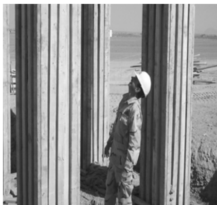
Don Hendrix, Tulsa District, inspects guard tower number 8's Formwork.
