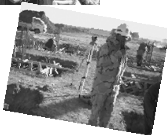
Ed Freer, DPW, Fort Campbell, inspecting the DFAC footer placements.
