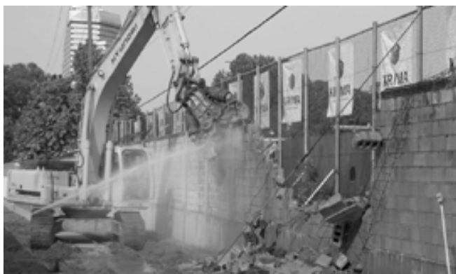
The backhoe with ripper jaws is tearing down the wall between Yongsan Garrison and Ministry of National Defense compound.
