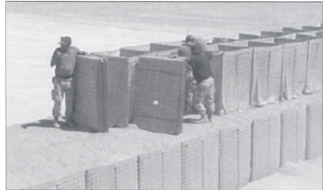
Example of HESCO wall construction
