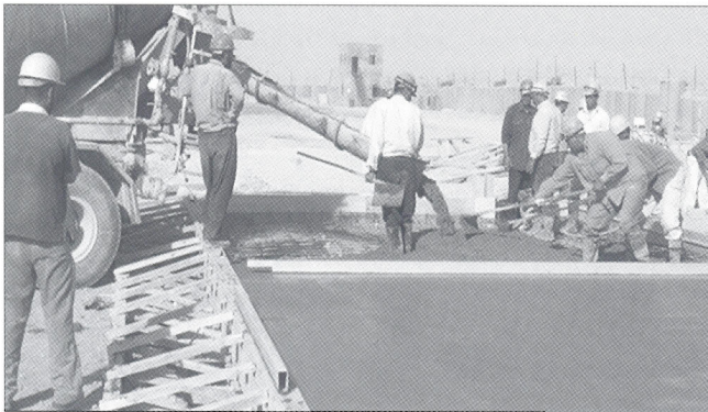
Pictured above is one of the slabs needed to construct the temporary camp. This particular slab is for a prefabricated metal housing unit.
