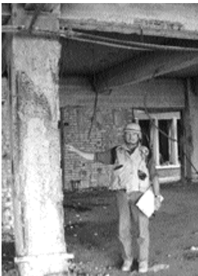
Mr. Flint provided a structural engineering assessment of a burned out government building (HQ Commission of Electricity).
