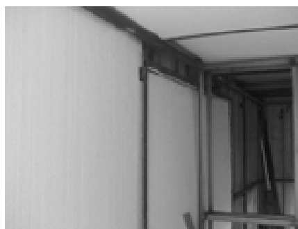
J2 OGA interior wall with sound abatement: One SCIF security requirement was 1 1/2 inch sound abatement material had to be placed between the exterior walls and the interior walls.
