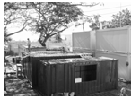
Level one placed with one for two being prepped: The first level of the SCIF is in place and the first container for the second level is being transformed into an office prior to being set atop the first level.
