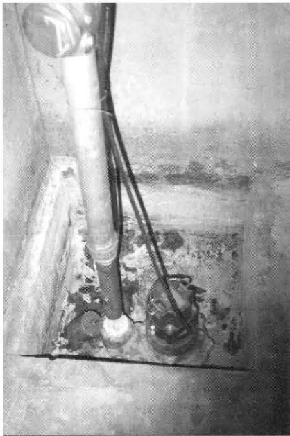
Some of the rust and deterioration in one of the underground areas evaluated for EOP technology to prevent additional damage.
