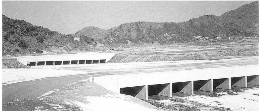
Two of five reinforced concrete culverts constructed as part of the Phase I work at the multipurpose range complex upgrade at the Korea Training Center. They were built as a flood control measure.
