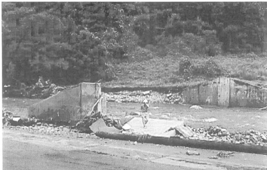
Mr. Chon, Kyong-Ho, FED electrical engineer, surveys damage to foot bridge abutments on Camp Hovey, as part of the flood recovery effort.
