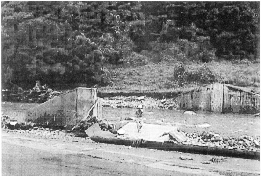
Mr. Chon, Kyong-Ho, FED electrical engineer, surveys damage to foot bridge abutments on Camp Hovey.
