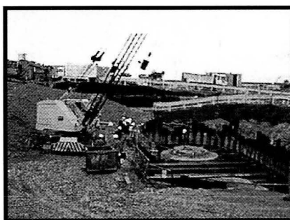
Open caisson excavation showing sheet pile bracing and two existing concrete piers to be incorporated into the completed foundation.
