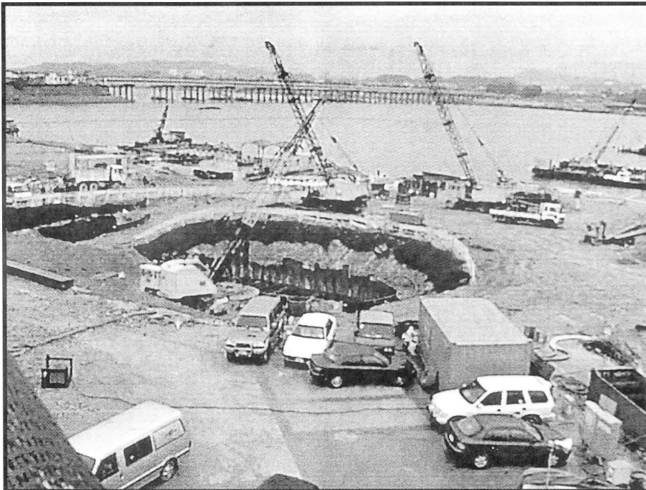
View of open caisson excavations along the northern Tangsan Bridge approach and in the Han River.
