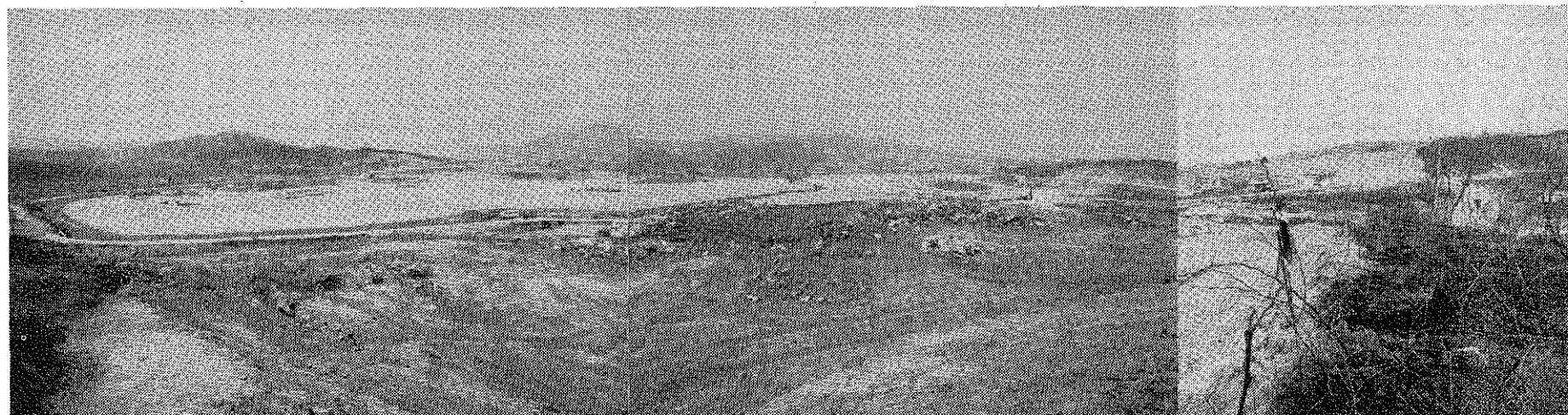
Approximately 650,000 cubic meters of earth have been moved in the first phase of the creation of a helicopter base located in Wonju next to Camp Long. Shown in this photo is the entire project as viewed from a nearby hillside.
