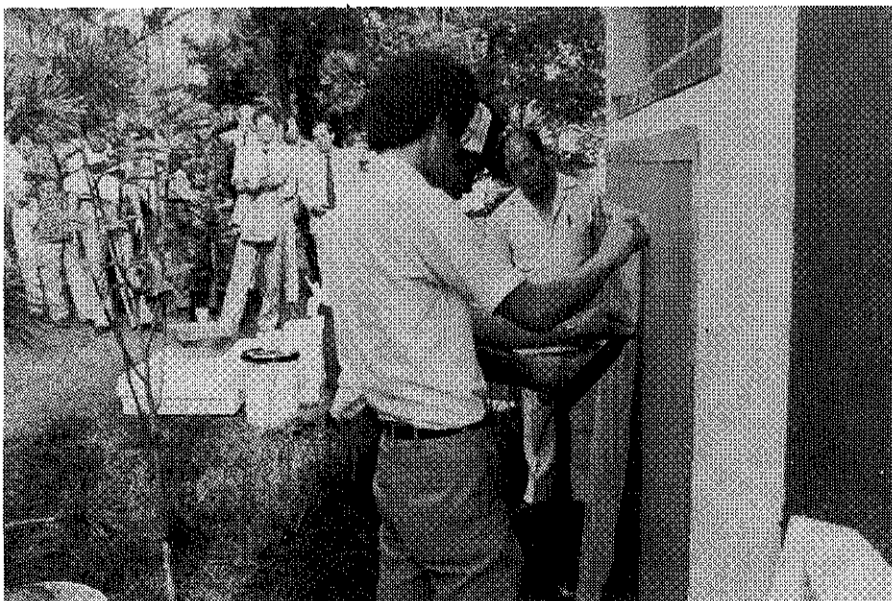
Exterior Insulation System A demonstration at FED.
