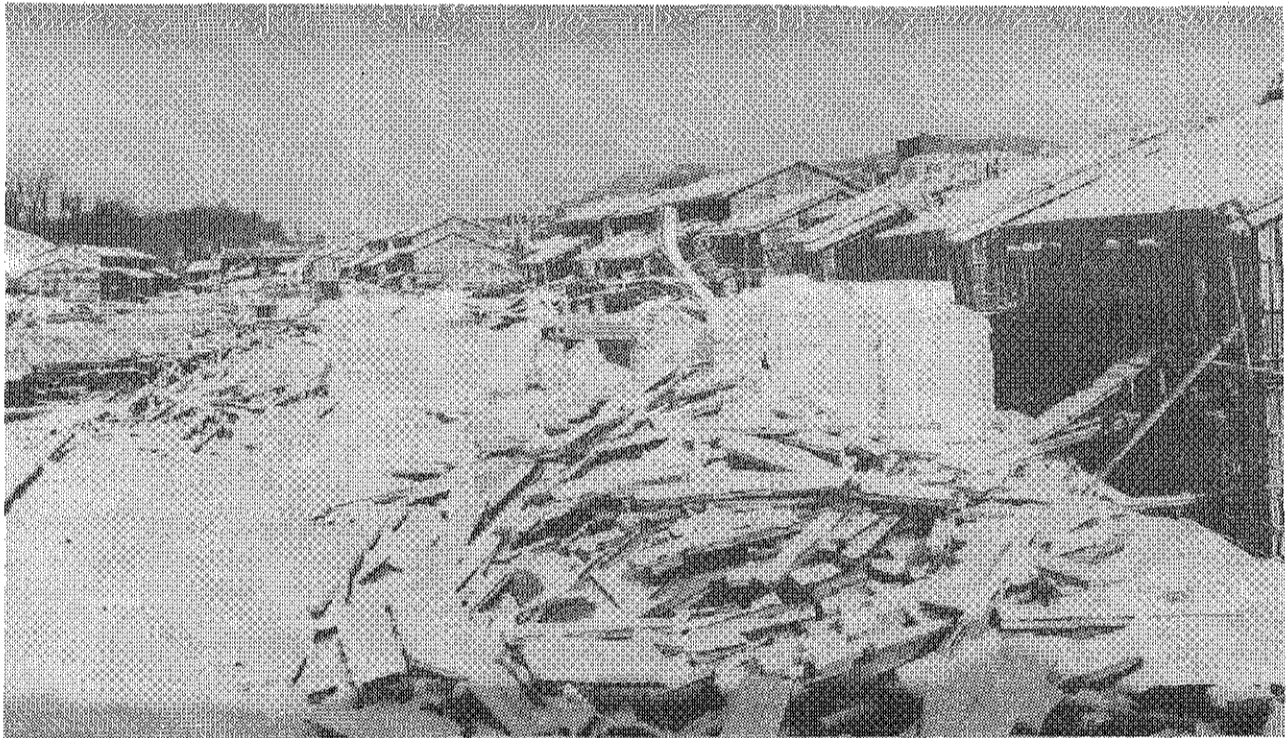
New Yongsan post housing under construction. A total of 300 housing units will be completed this summer by the Korea National Housing Corporation, replacing the current RGH family housing. This special project places FED in a surveillance role rather than a quality assurance role it normally provides customers.
